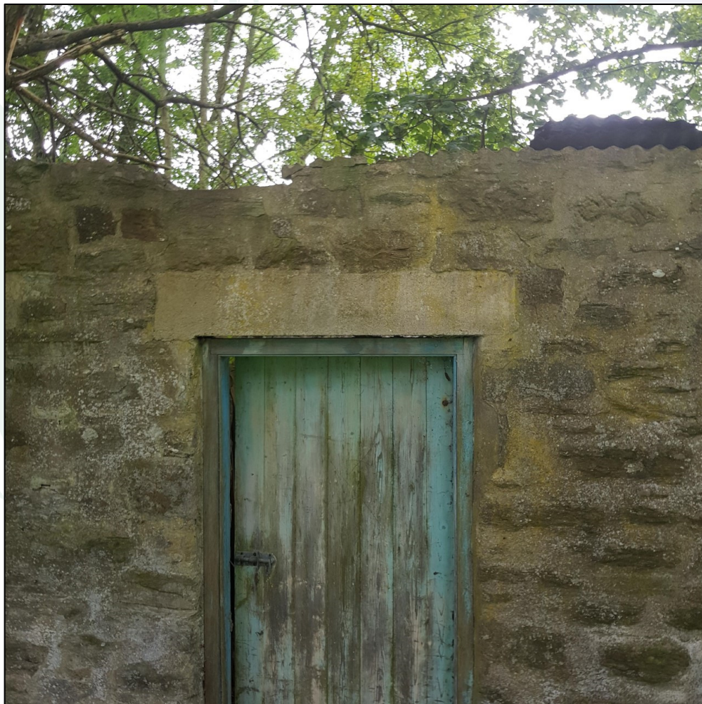
Figure 2. Front of building.
