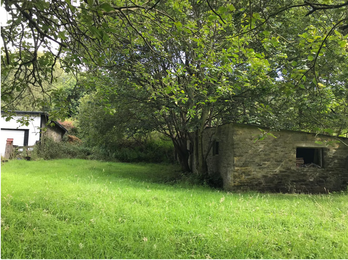
Figure 4: Dilapidated Bleach Works Building
