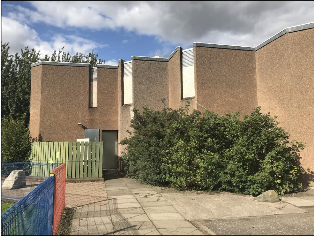
Figure 3 – South West Corner of Lochside Leisure Centre
