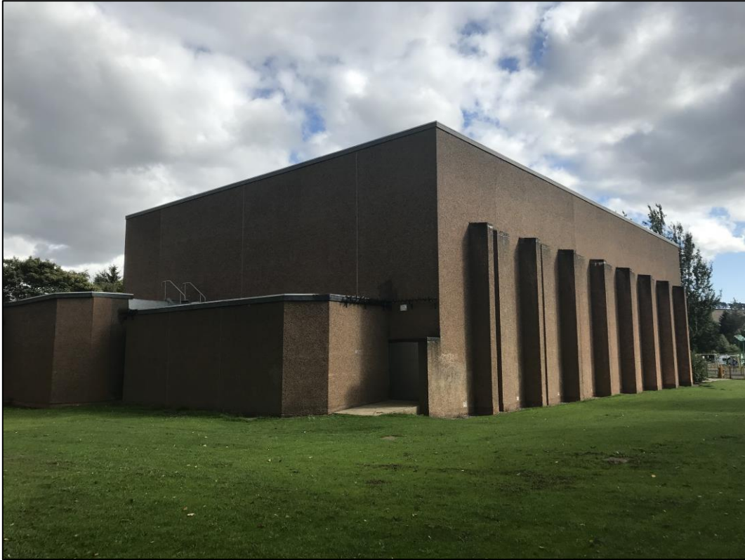
Figure 7 – North and West Elevation of Sports Hall showing Single Storey Storage Area
