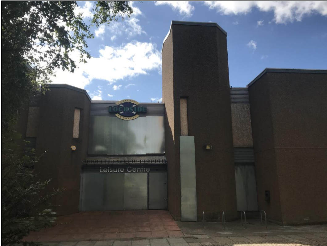
Figure 1 – Front (East) Elevation of Lochside Leisure Centre
