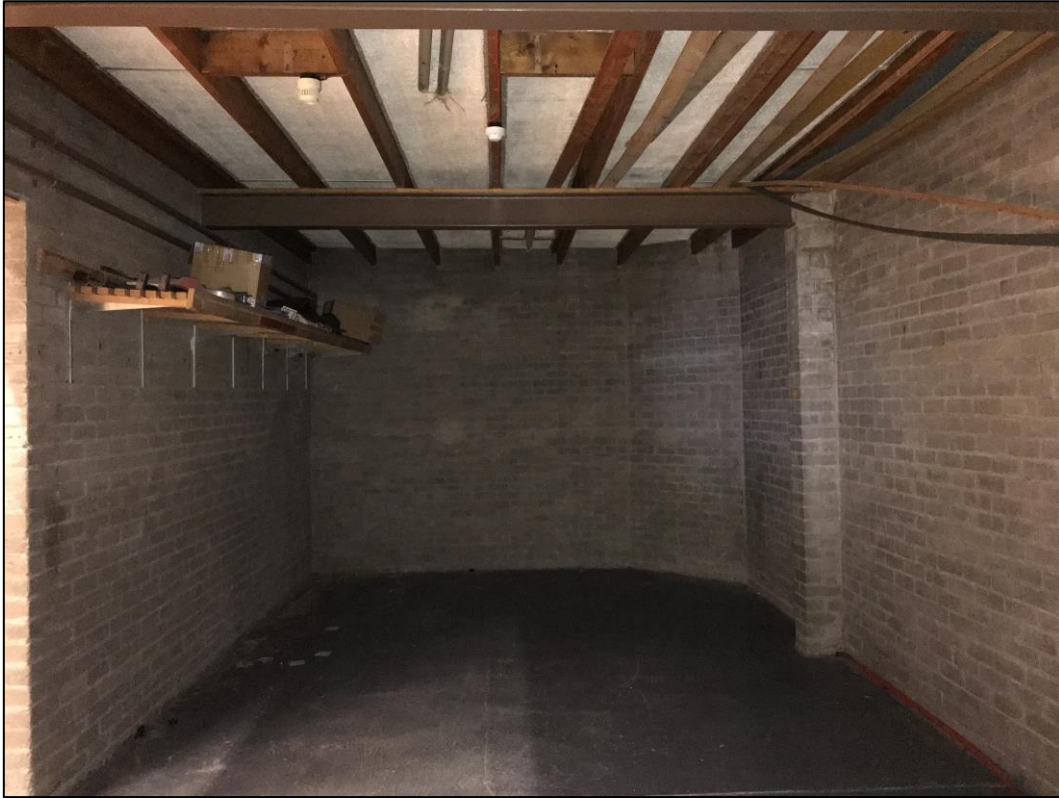
Figure 11 – Internal Structural Arrangement of Sports Centre Store
