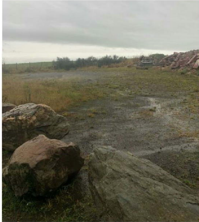
Views across site with hard core surface evident
