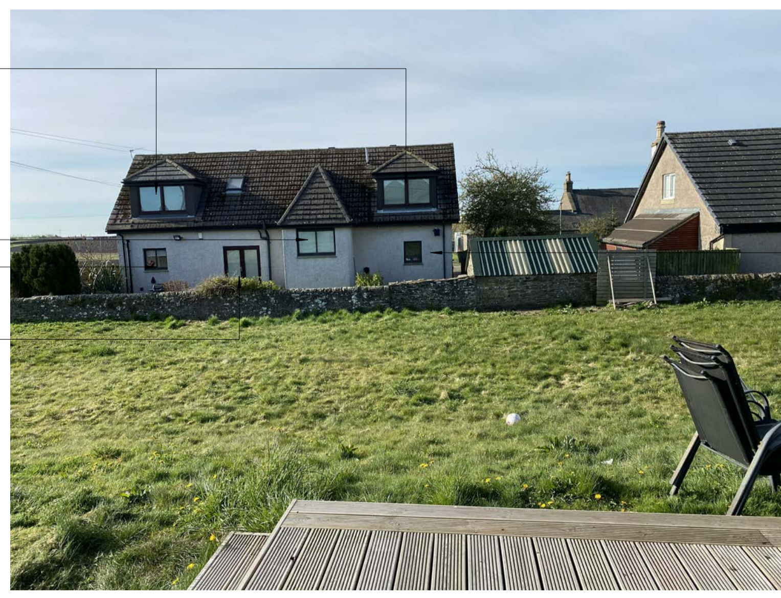
IMAGE C - 34A PITAIRLIE ROAD HOUSE ELEVATION LOOKING NORTH TOWARDS NEW PLOT
