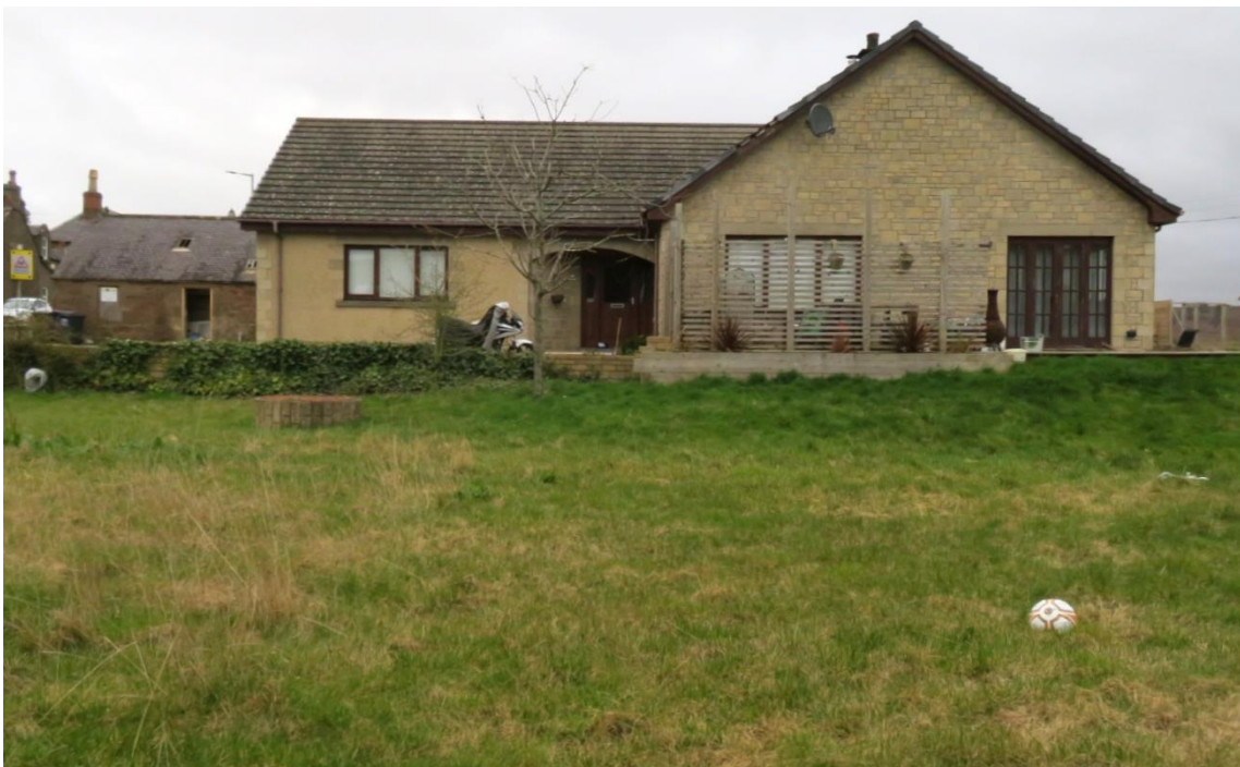
View of No. 32 from No. 34's kitchen dining room window after the appellant removed all pre-existing shrubbery planted by the previous owner to provide privacy. This also shows the south facing windows of NO. 32 that would have to be removed if the plan were approved.
