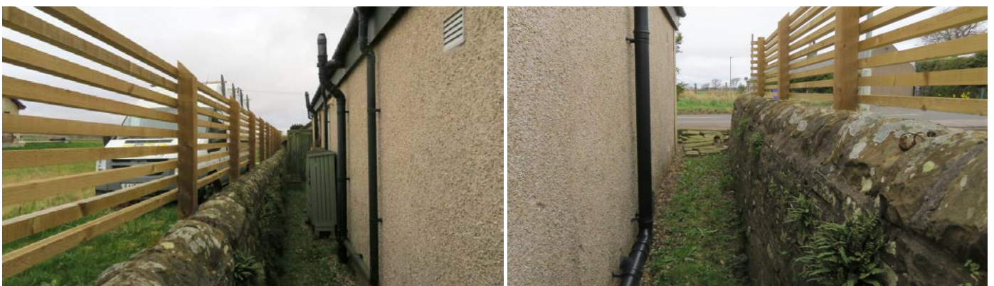
Views emphasising the artificial height difference between the plots, which used to not exist, and how much lower than the road No. 34 is set.
