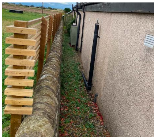
Boundary with 34 Pitairlie Road, demonstrates the level difference, existing wall and fence
