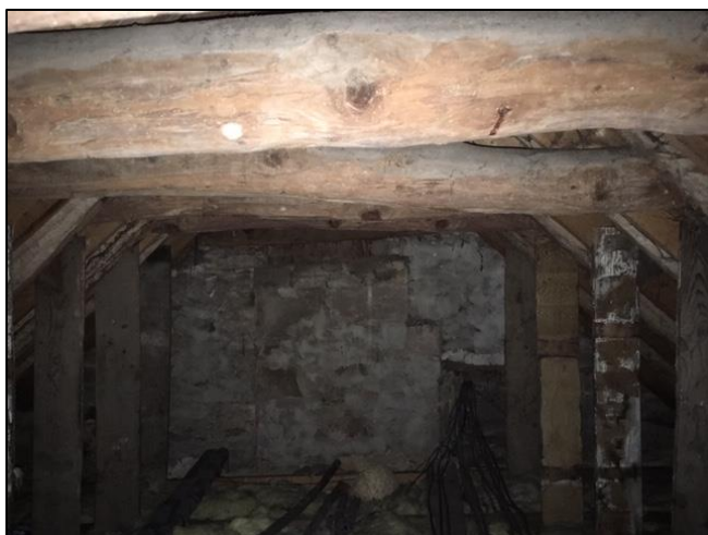
Photo 7: Inside main attic space of bungalow
