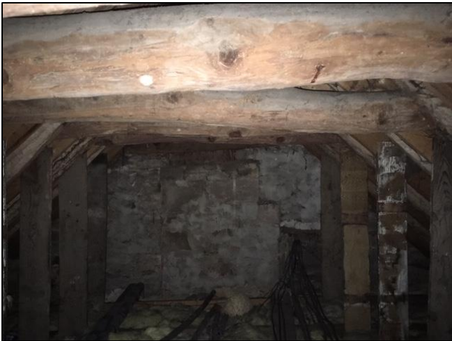
Photo 7: Inside main attic space of bungalow
