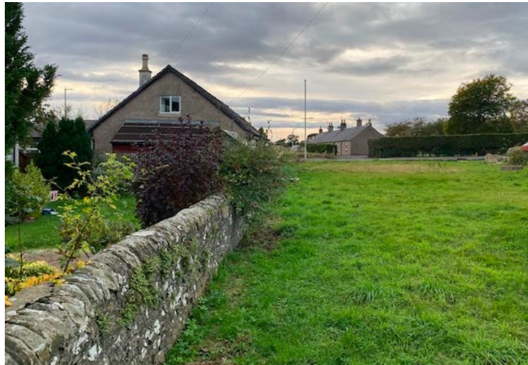
Existing wall along southern boundary of site
