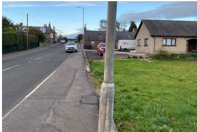
Road frontage, clear visibility in both directions
