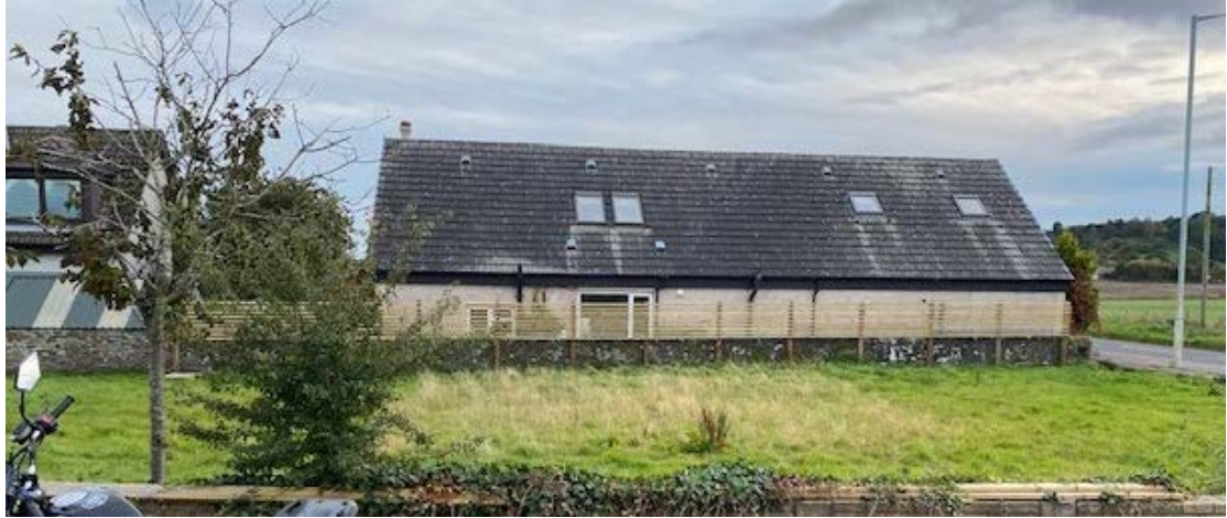
Rear elevation of 34 Pitairlie Road, house set lower than appeal site, kitchen window already compromised by northern elevation, level difference existing wall and fence. Window currently overlooks front garden area of 32 Pitairlie Road
