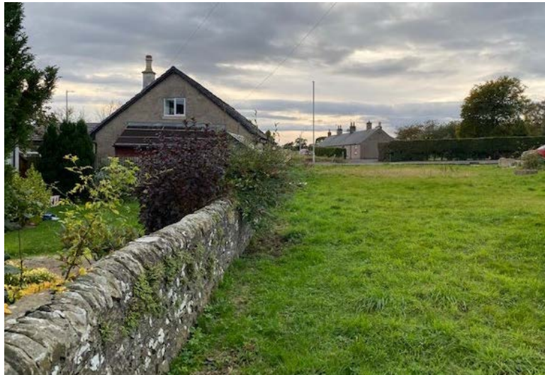
Existing wall along southern boundary of site
