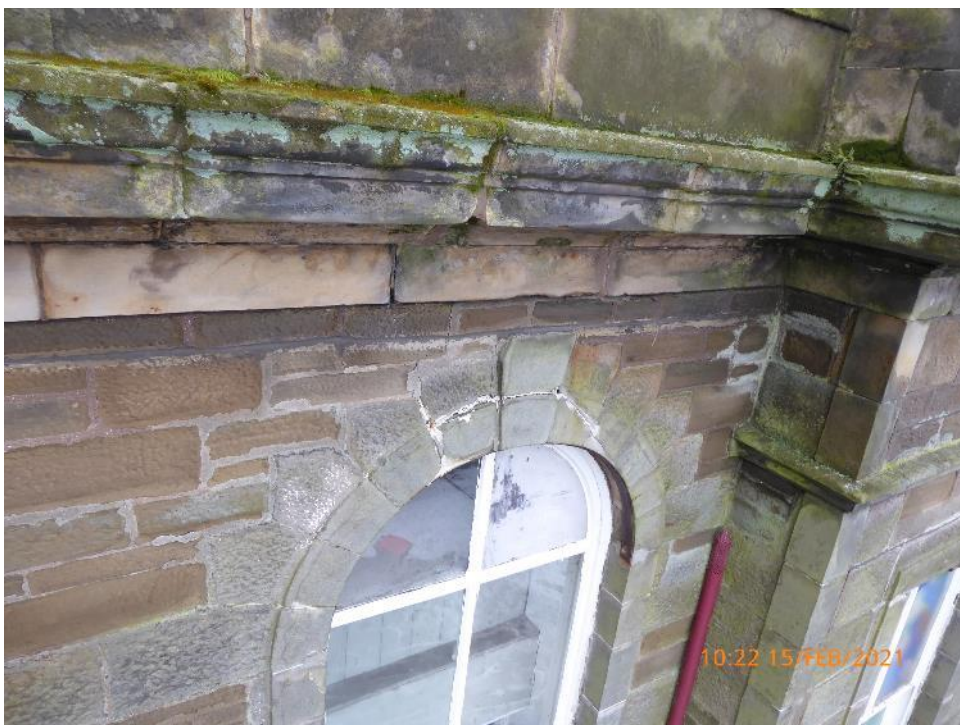
10. Erosion and missing pointing
