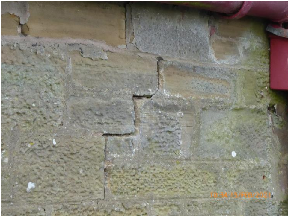
13. Cracking to east elevation
