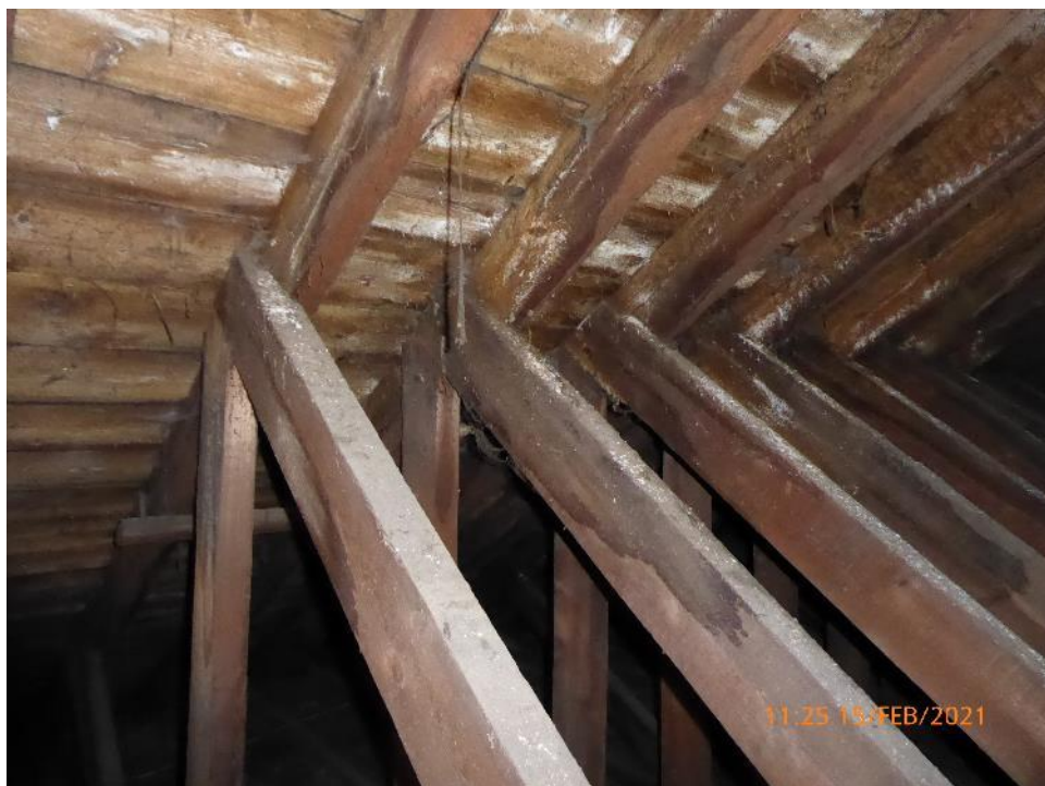
29. Water staining of roof timbers
