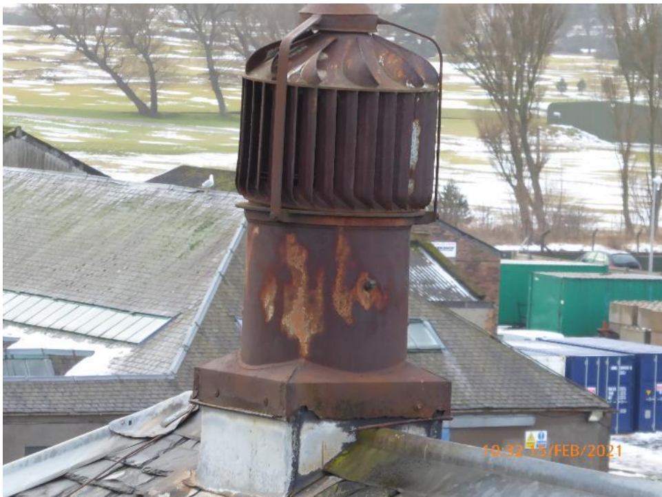
27. Heavily corroded roof vent
