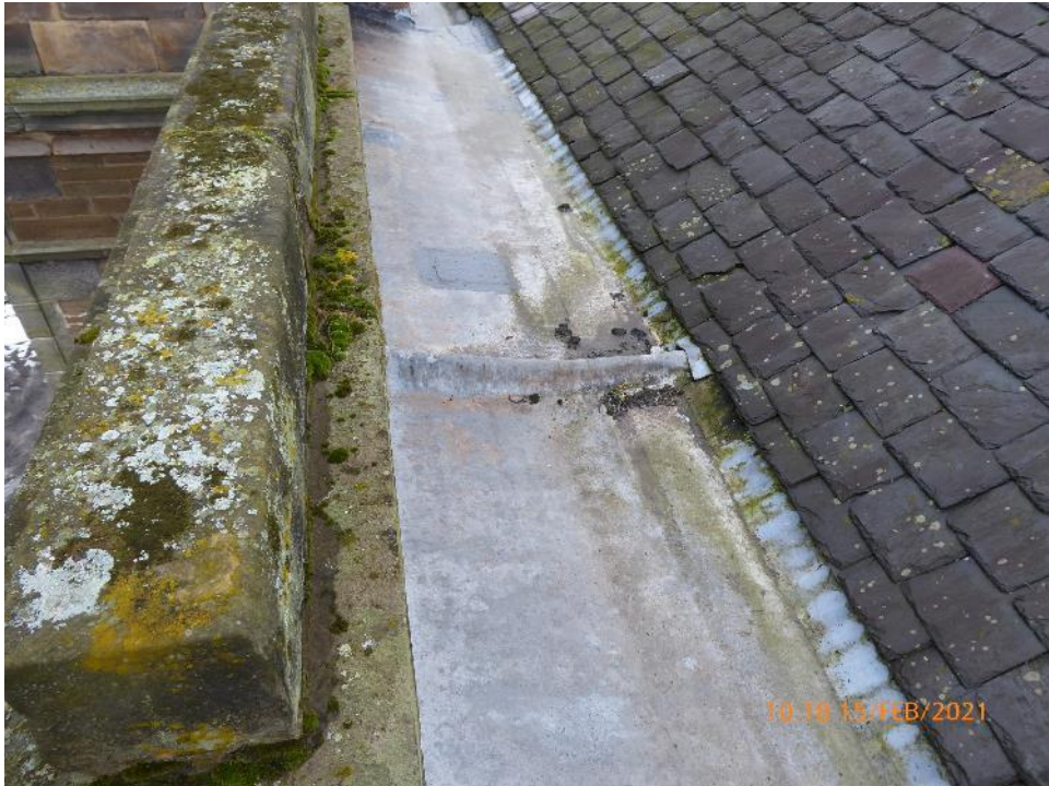
21. Patch repairs to lead
