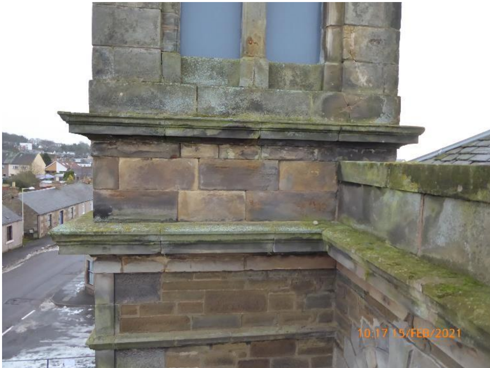
9. Erosion and missing pointing
