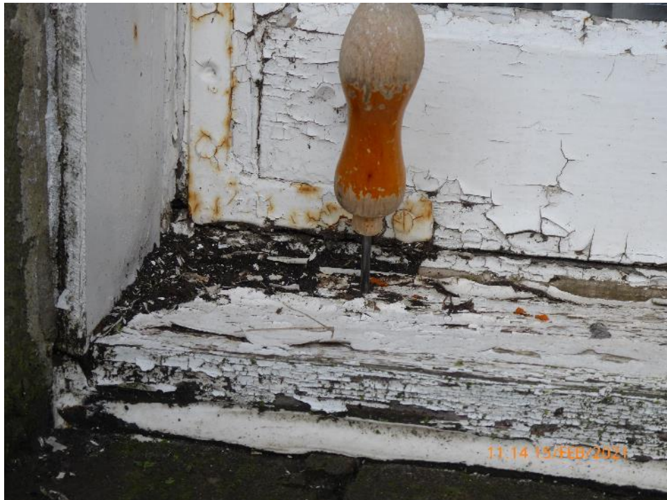
19. Decay (and previous patch repair)
