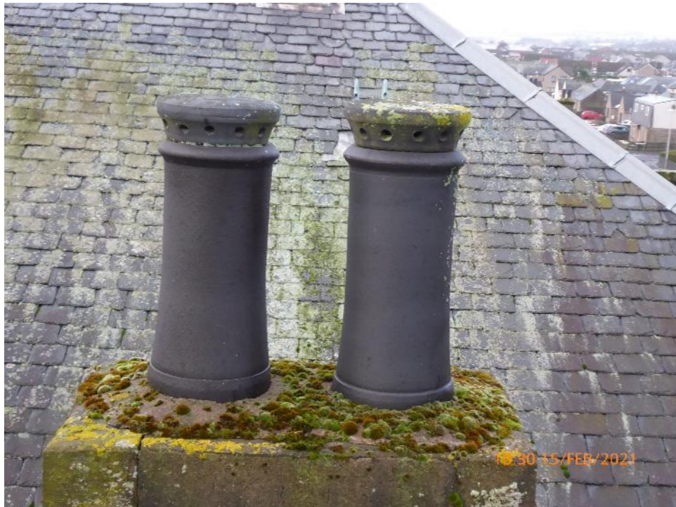
24. Cracking of flaunching
