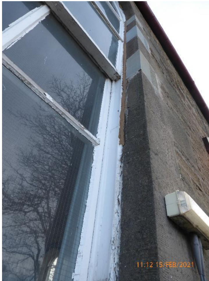
18. Loose/missing and dislodged pointing around window
