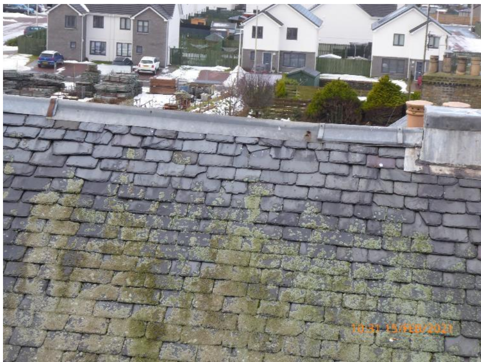
25. Loose, missing and dislodged slates
