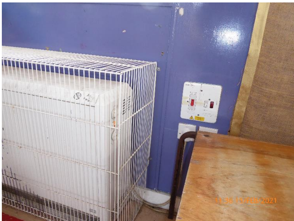
35. Aged electrical heating
