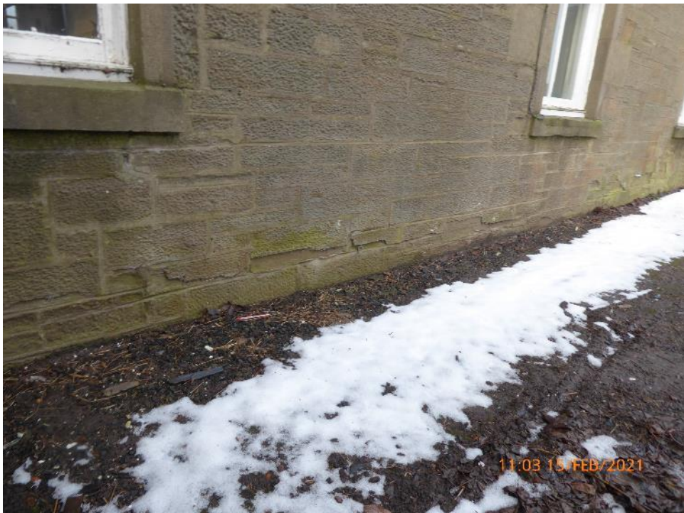
14. Typical low level erosion
