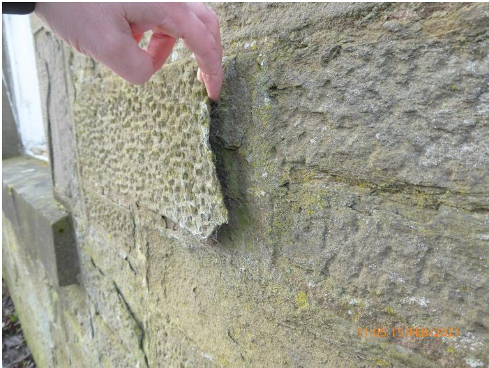
15. Typical scaling of stone
