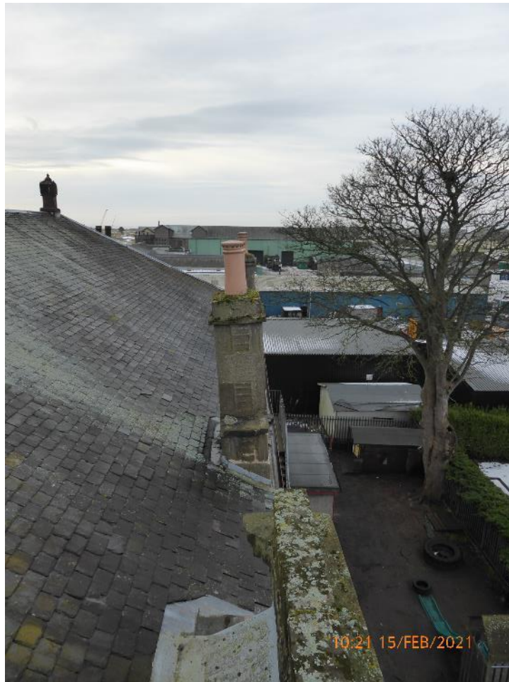
23. Typical leaning chimneyhead
