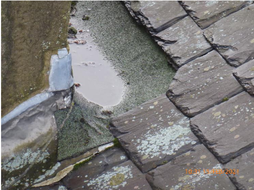
26. Temporary felt repair to rear of chimneyhead
