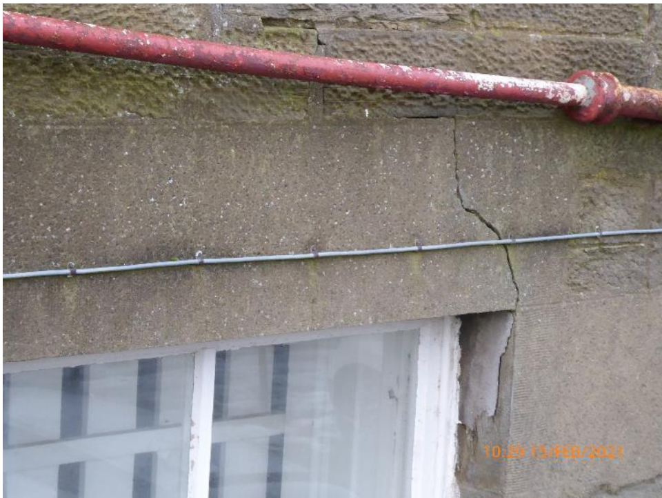
12. Cracking to head of window
