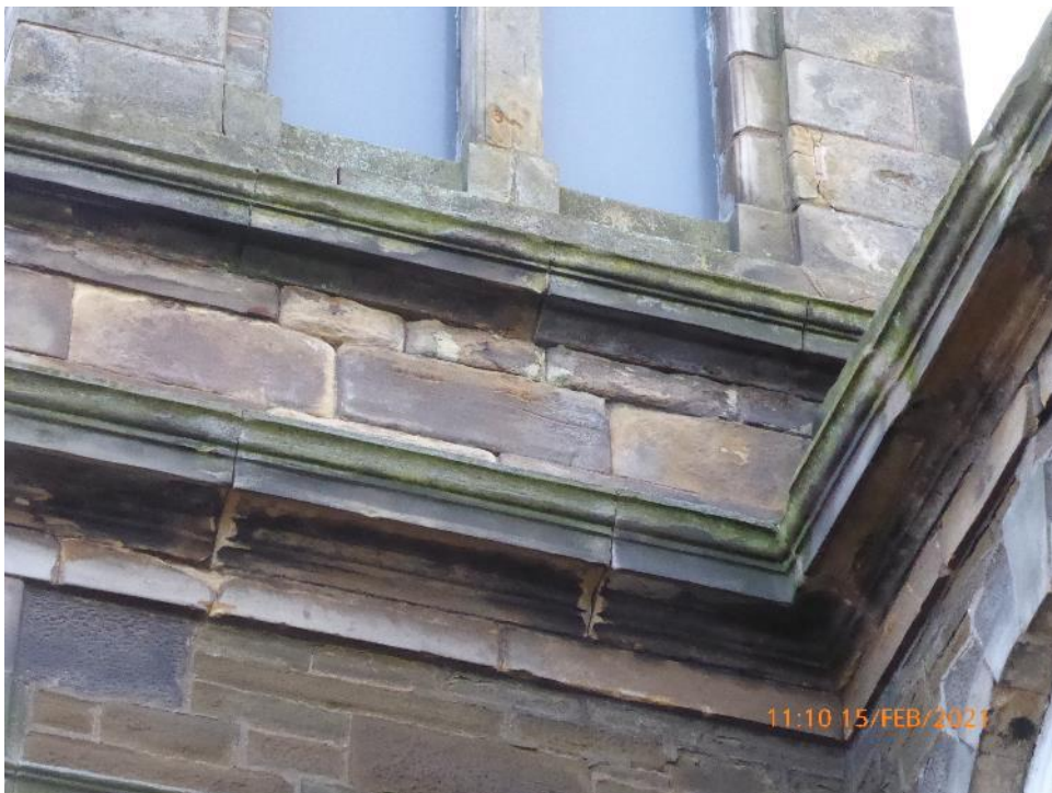
16. Erosion and missing pointing
