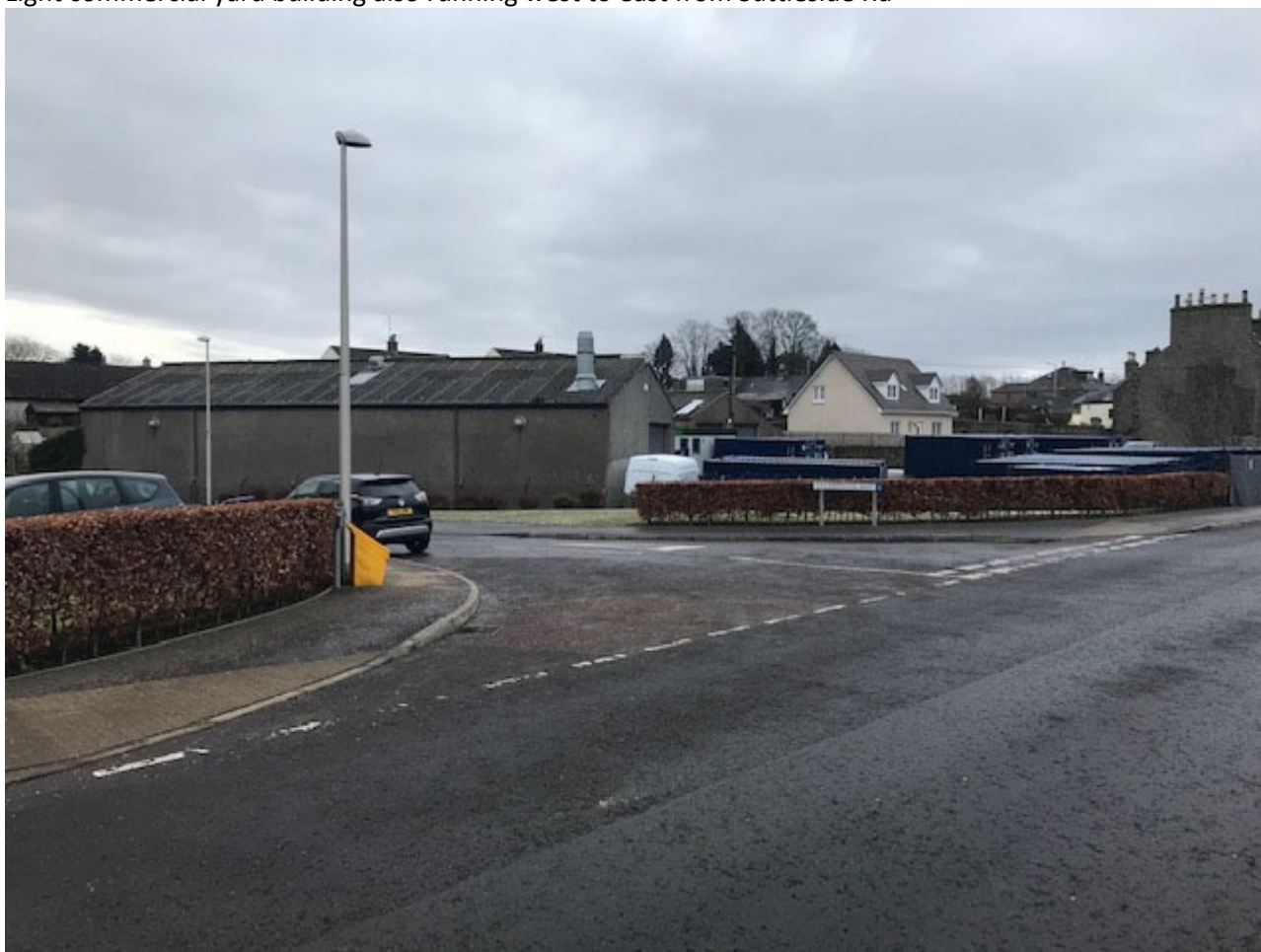
Light commercial yard building also running west to east from Suttieside Rd
