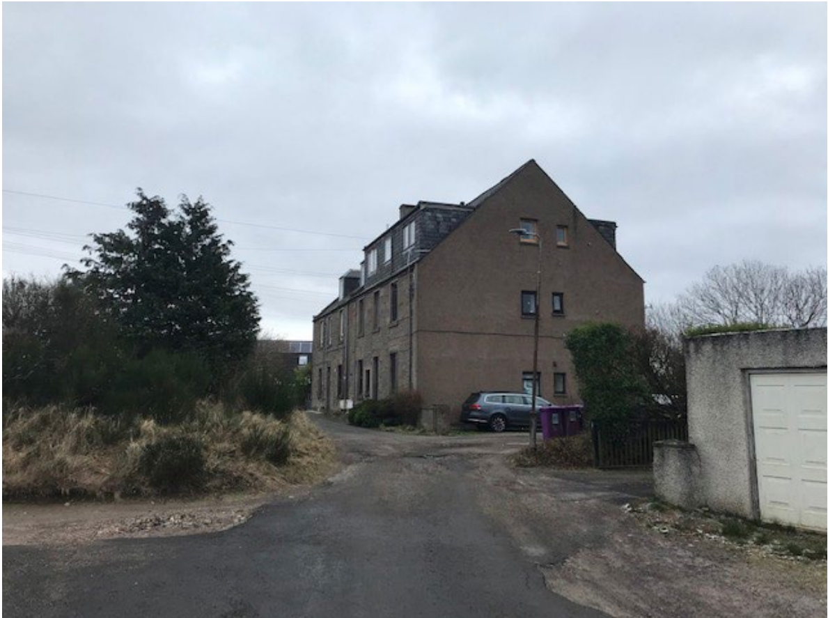
3 story tenement running west to east from Suttieside Rd along Alpha Place
