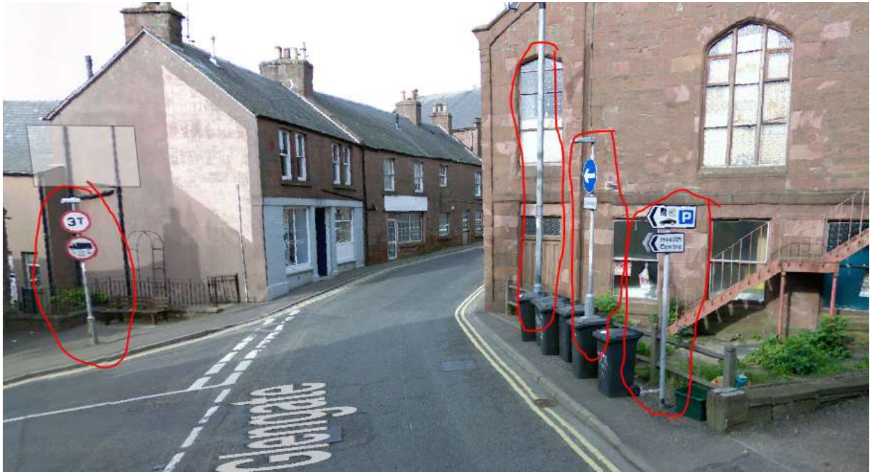
Image 5: Remove pole and signage to left. Rationalise signage on the right to be included on the one lamp standard. Lamp standard to be moved to where existing directional signage exists.
