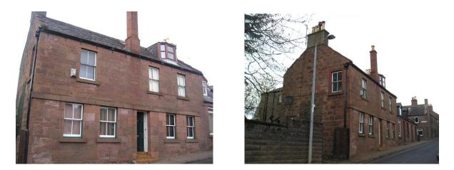
The grant eligible works comprise 1) stonework repairs to remove cementitious render, indent new stone where necessary and to repoint in lime mortar on all three elevations (90sq.m at front, 60sq.m to side and rear) including the front chimney; and 2) comprehensive repairs to 7no. traditional timber sash windows on the front elevation and 2no. on the gable
