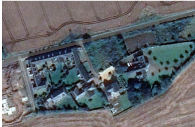
Aerial view of site, boundaries on all sites clearly evident
