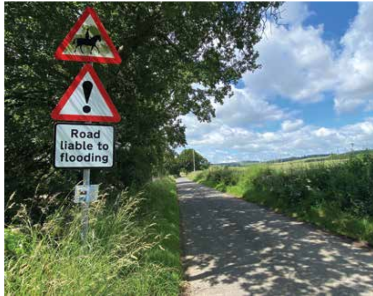
BERRYHILL ROAD IS ALREADY KNOWN AS A FLOOD RISK.
