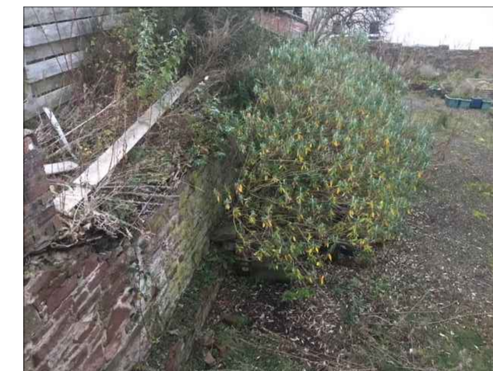
Existing retaining wall forming North Boundary.
