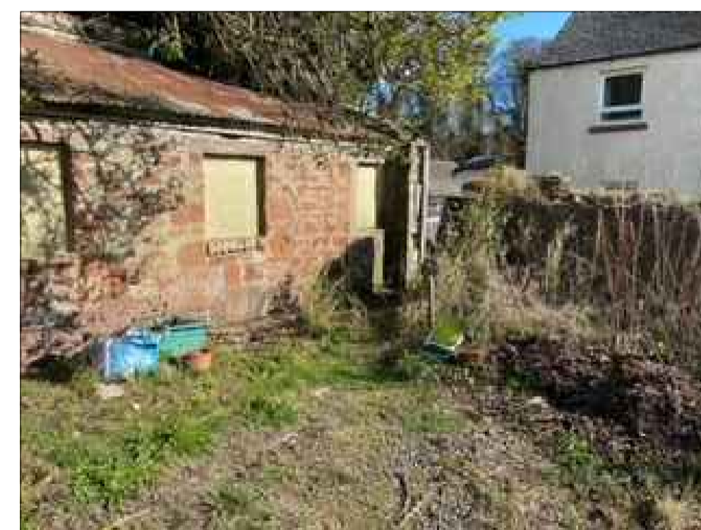
Existing derelict building on site
