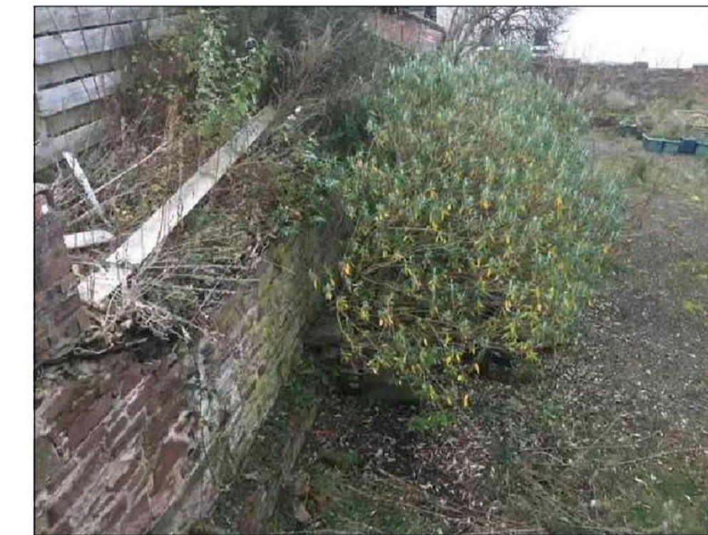
Existing retaining wall forming North Boundary
