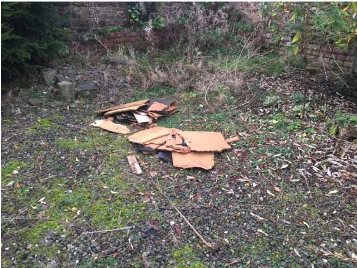
The foot print of the former Church Hall is predominantly hard standing covered with gravel and encroaching vegetation.
