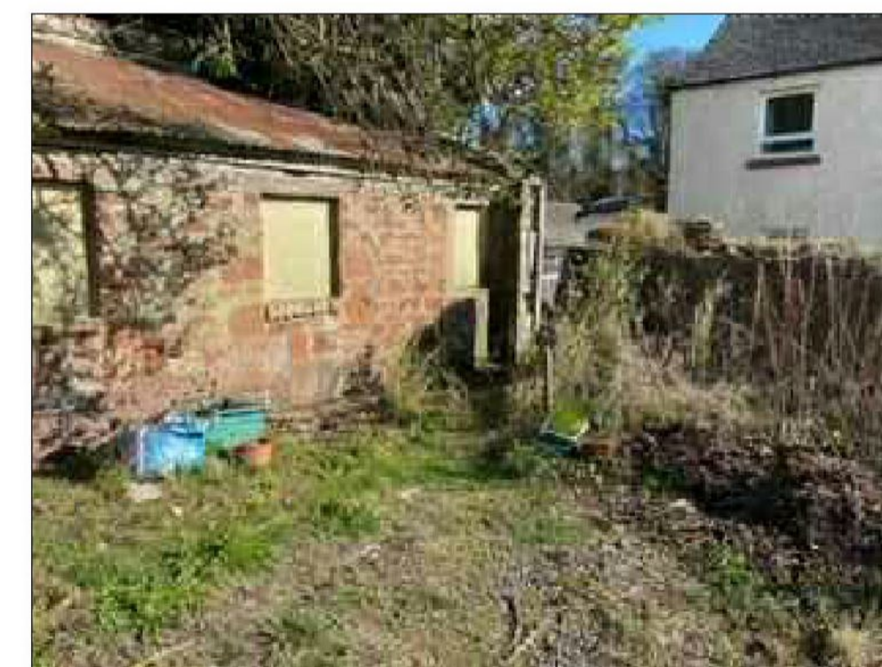
Existing derelict building on site
