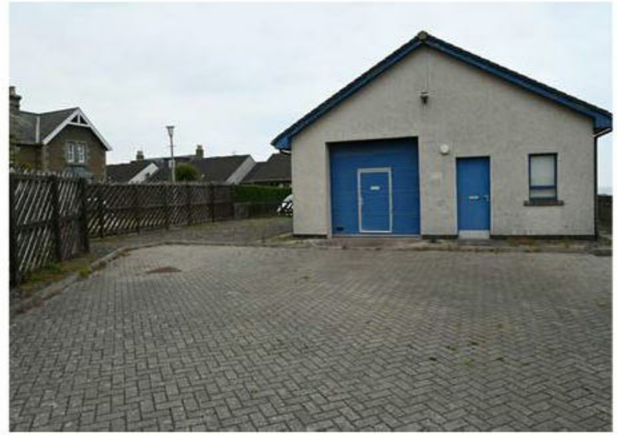
Coastguard Station & existing boundary
