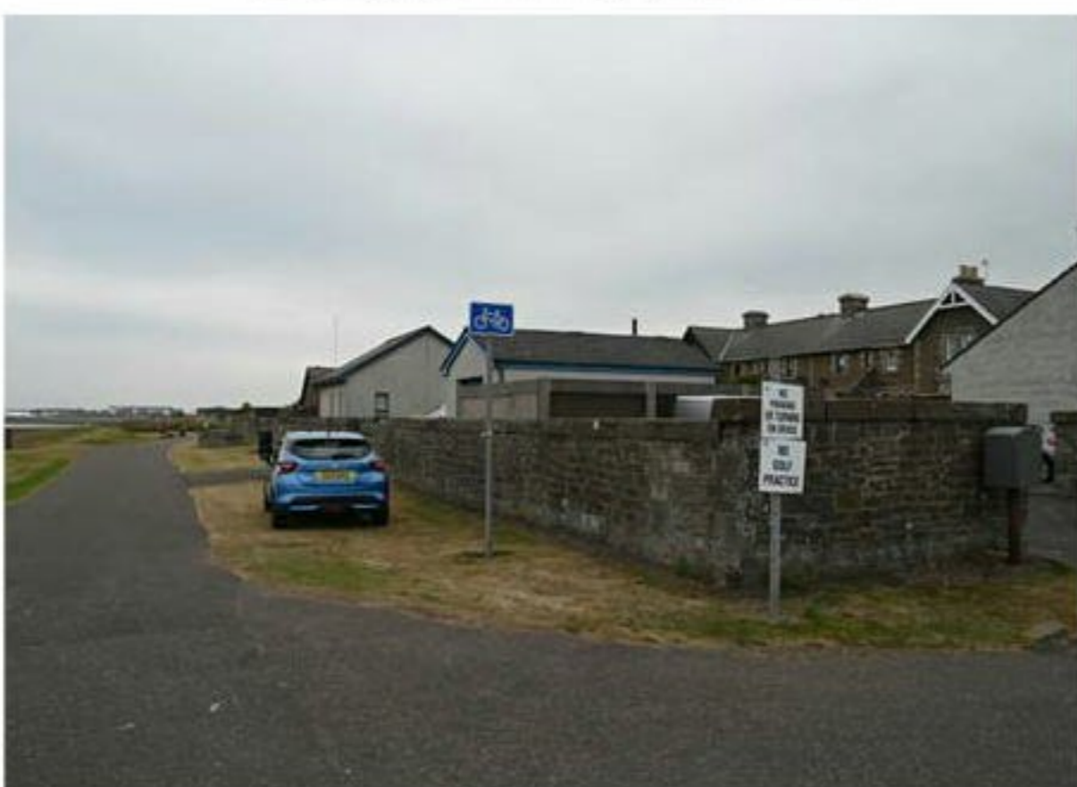
Existing cycle route and out buildings at East of site
