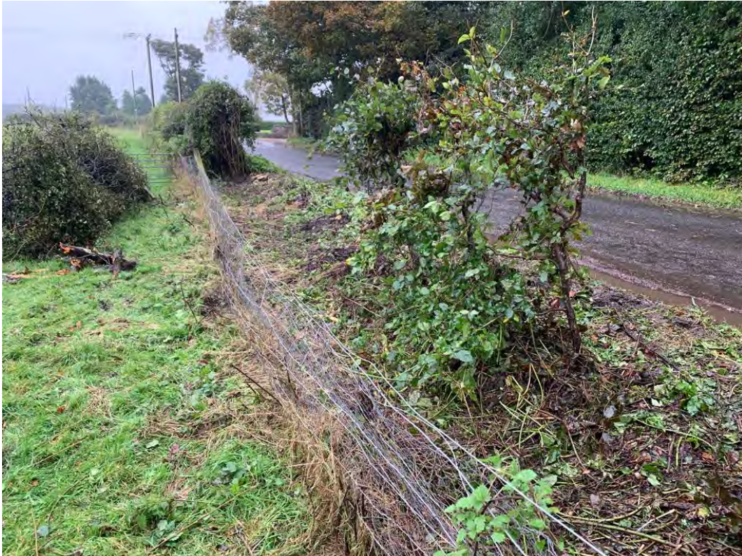
Figure 3: The combined 20m long damage from Accidents 1 & 2 to the hedgerow and stock fencing.
