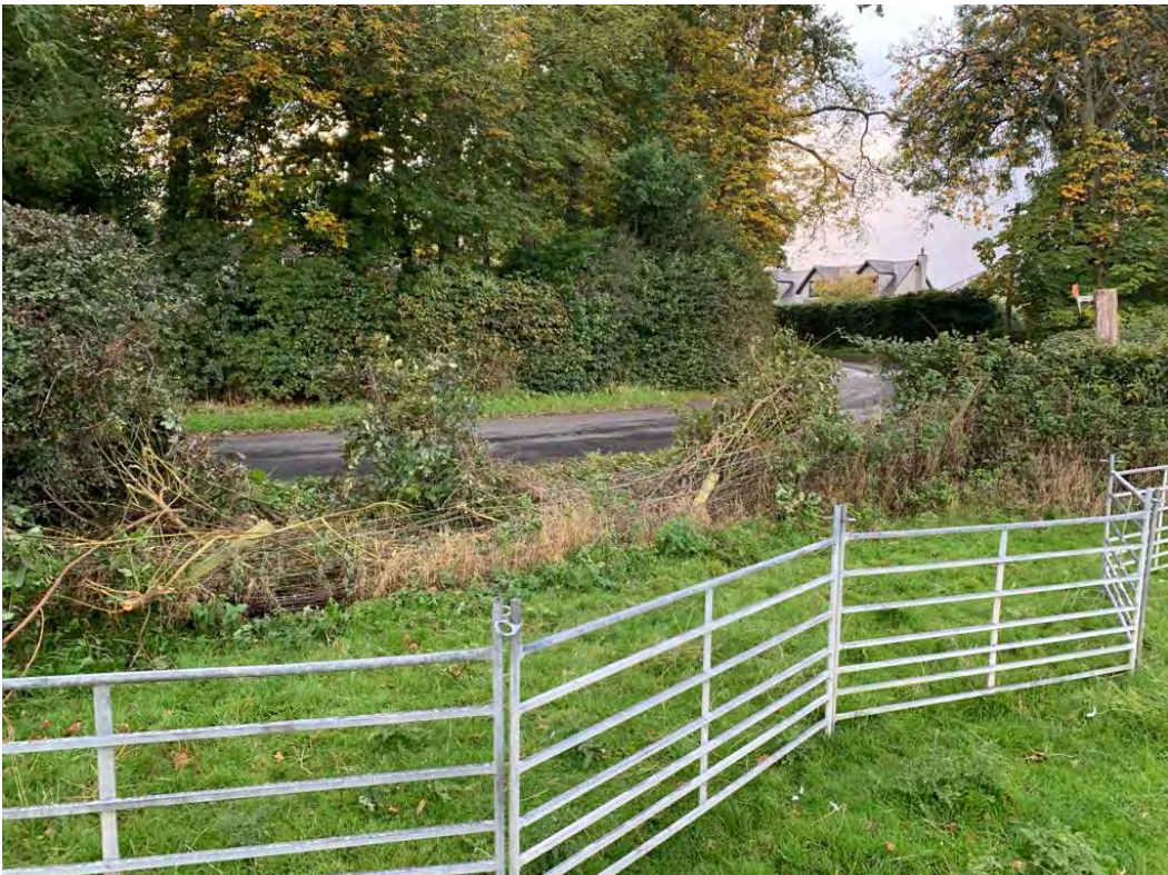
Figure 2: The 12m long damage from Accident 1 to the hedgerow and stock fencing.
