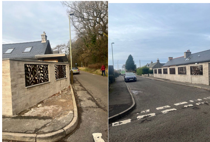
Existing unfinished wall
