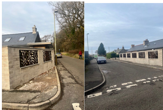
Existing unfinished wall
