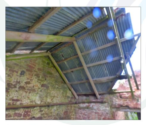
Figure 4. Corrugated sheet construction at rear.
