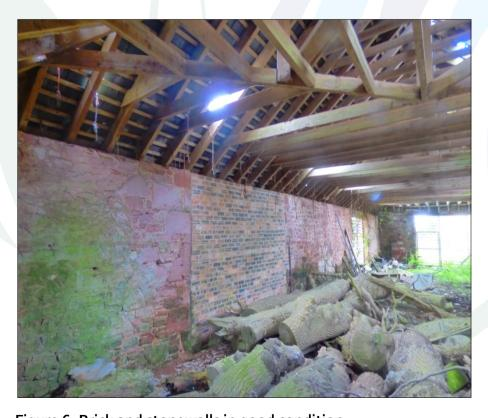
Figure 6. Brick and stonewalls in good condition.
