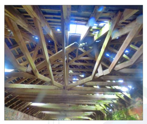
Figure 5. Slates on batons with numerous holes.
