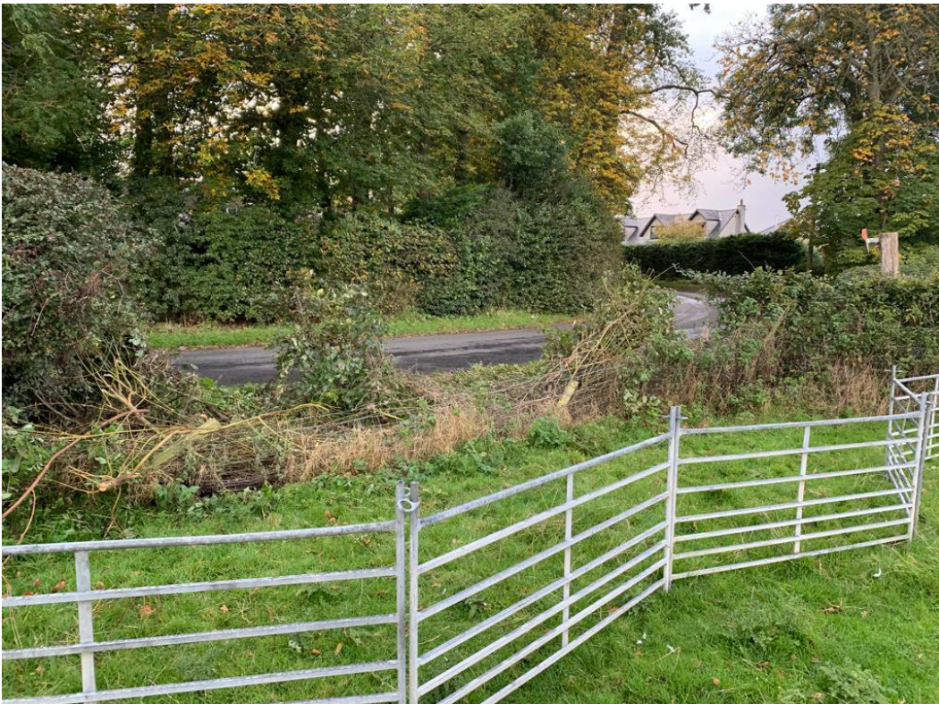
Figure 2: The 12m long damage from Accident 1 to the hedgerow and stock fencing.
