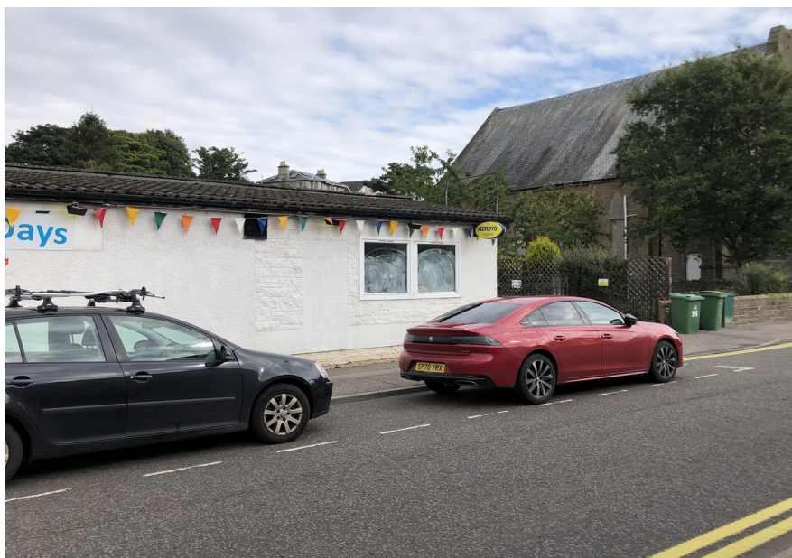
Existing South Elevation facing Dundee Street
