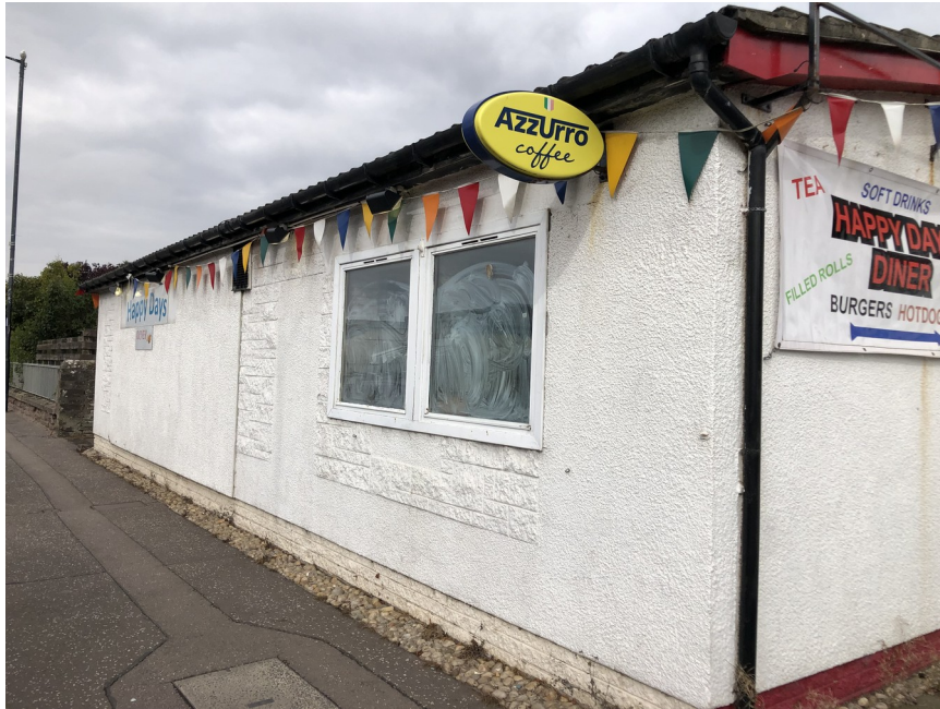
Existing South Elevation from the East.
