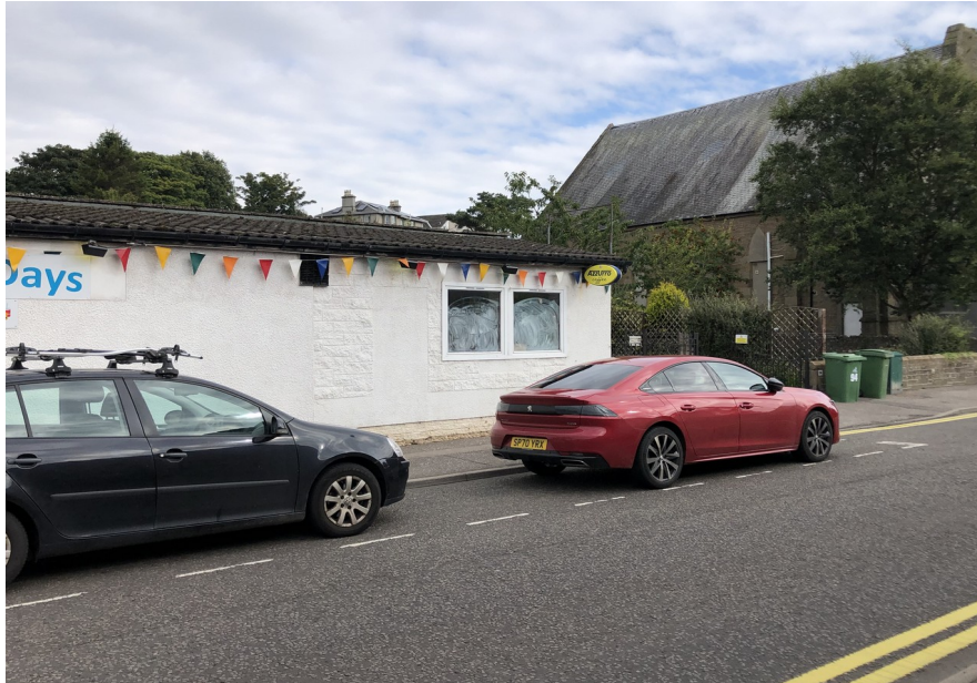
Existing South Elevation facing Dundee Street
