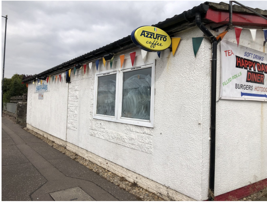
Existing South Elevation from the East.
