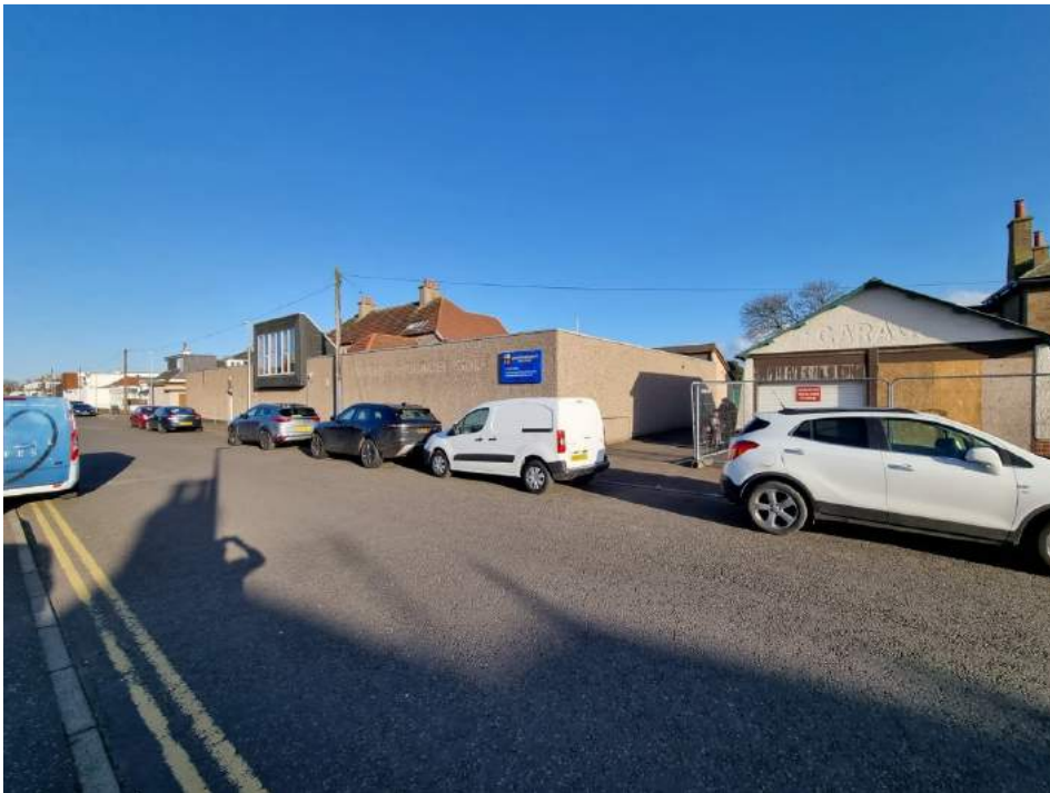
Figure 5 – Application site from Princes Street.
