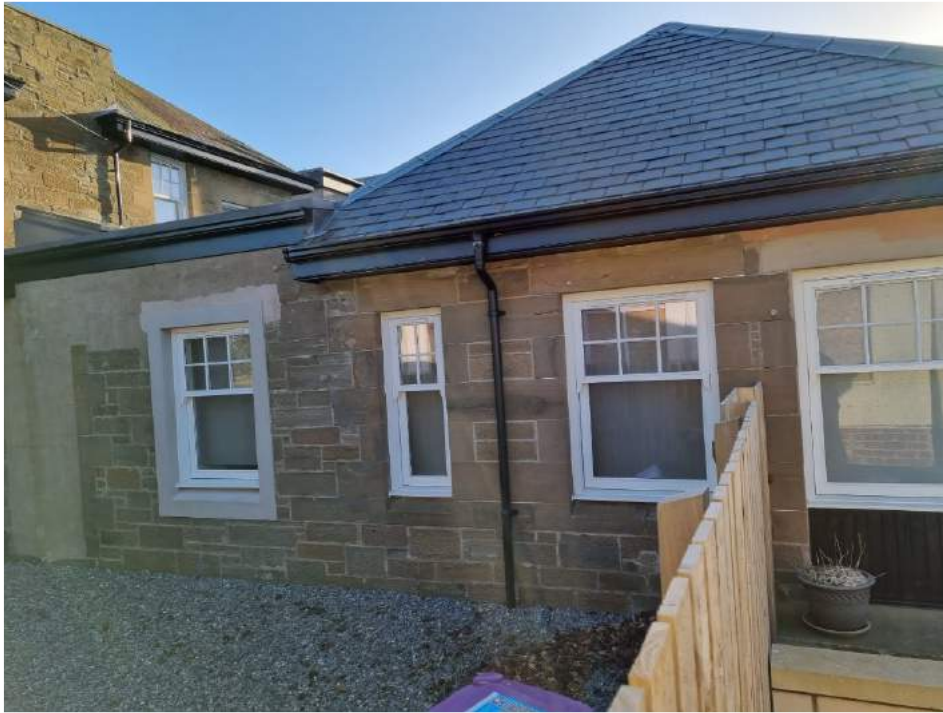
Figure 6 – Previously converted property at former Panmure Hotel.
