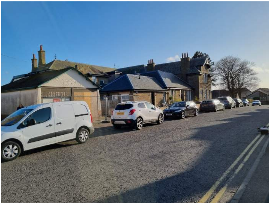
Figure 7 – Application site from Princes Street.
