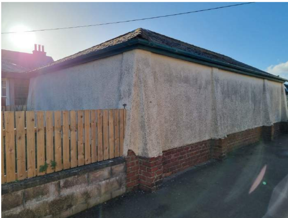
Figure 21 – Side of application site.
