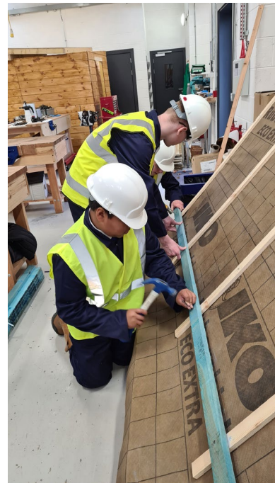
S3 Foundation Apprenticeship pupils preparing a roof for tiles.
