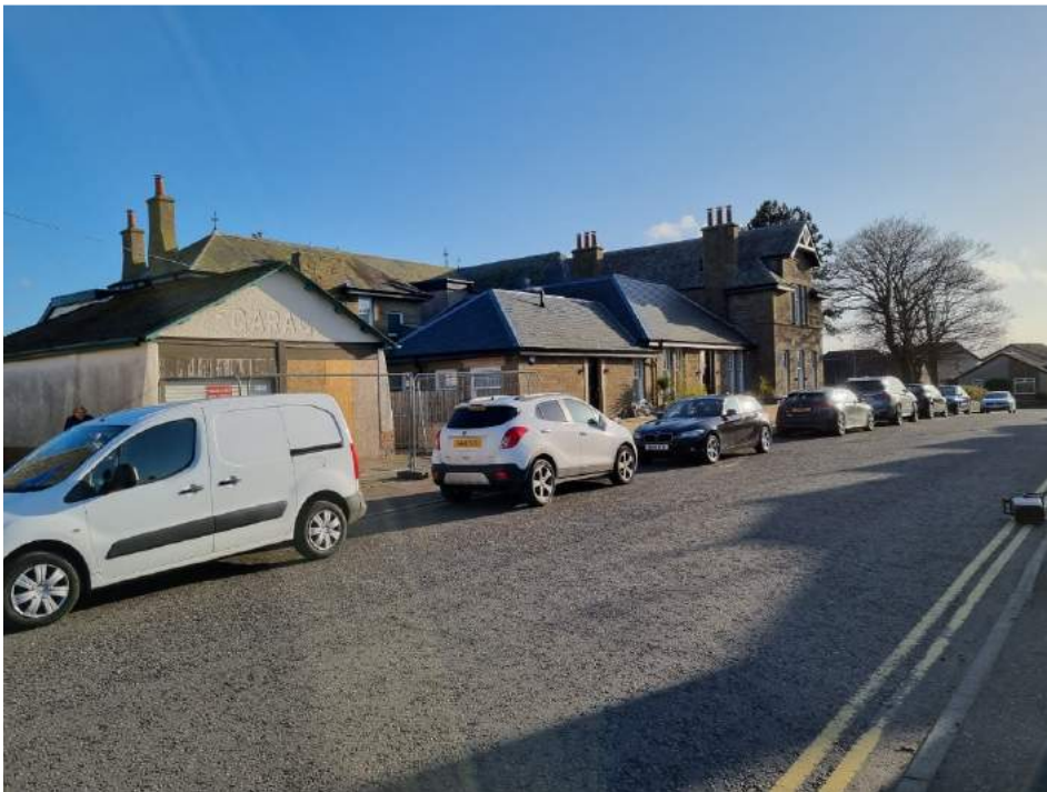
Figure 7 – Application site from Princes Street.
