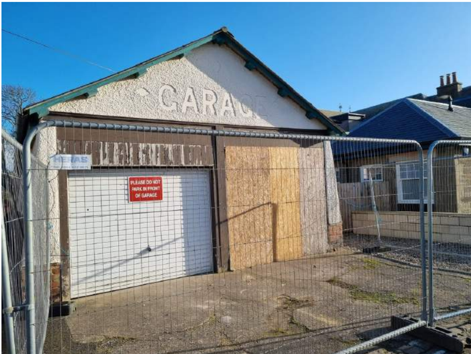
Figure 23 – Front of application site.
