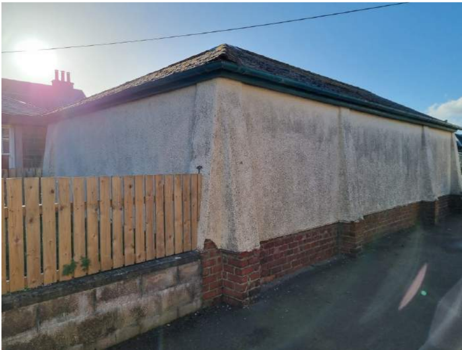
Figure 21 – Side of application site.
