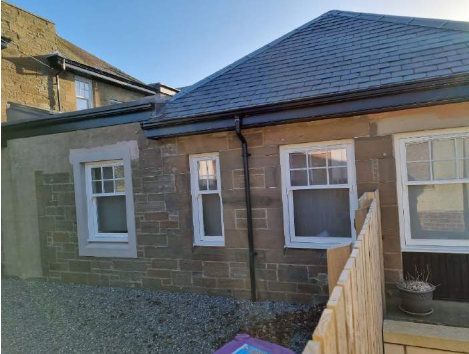
Figure 6 – Previously converted property at former Panmure Hotel.
