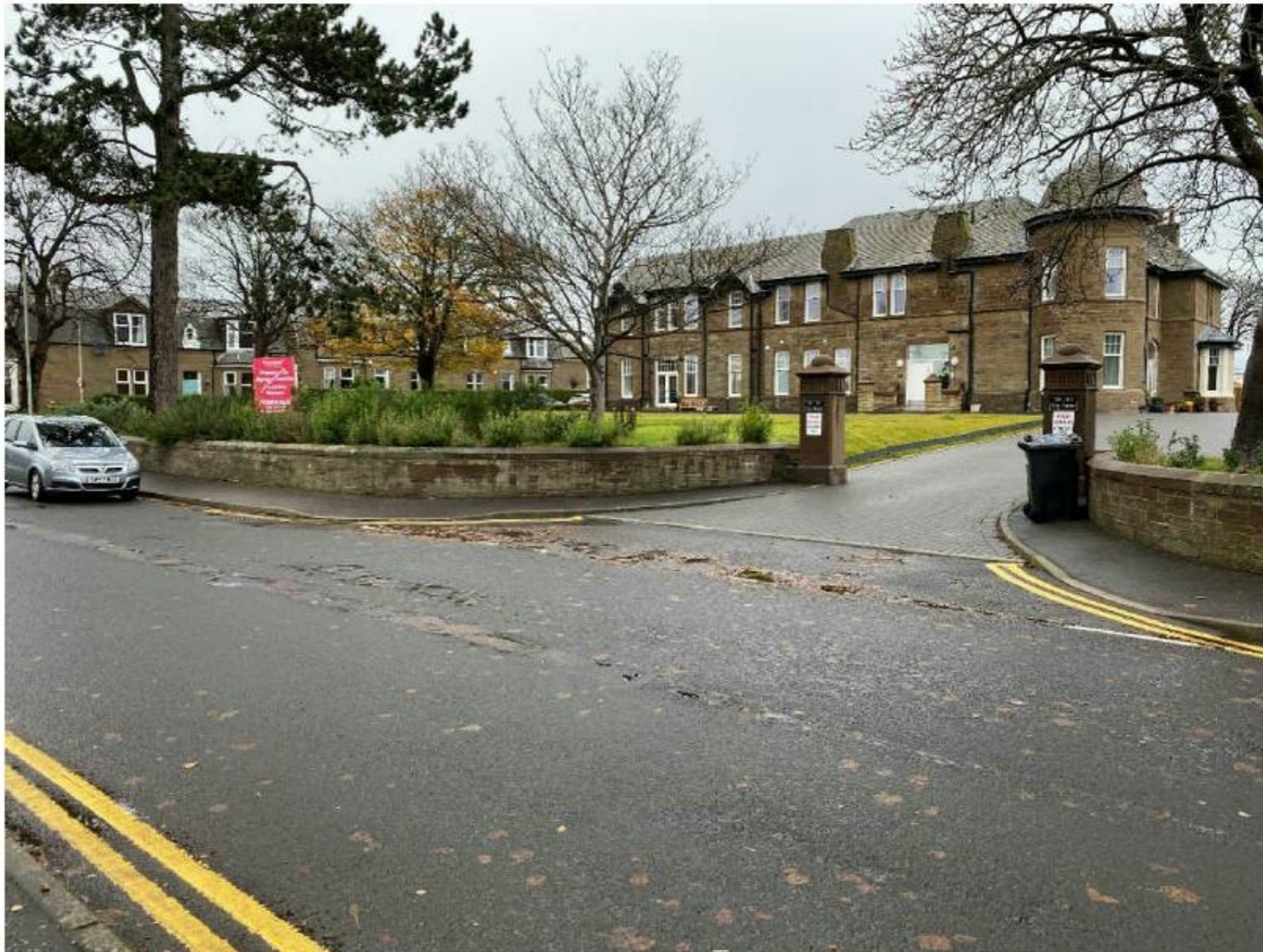
Photographs 1 – Looking north eastwards towards the site from Tay Street. The site extends across the grassed area in the centre of the photograph. As can be seen the site sits significantly higher than Tay Street. The top of the masonry boundary wall is approximately 0.9m to 1m above the back of the footway in the vicinity of the large tree in the top left of the photograph.
