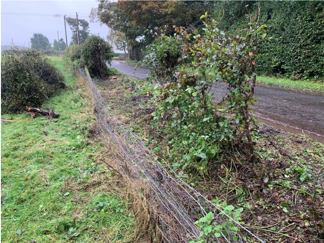
Figure 3: The combined 20m long damage from Accidents 1 & 2 to the hedgerow and stock fencing.
