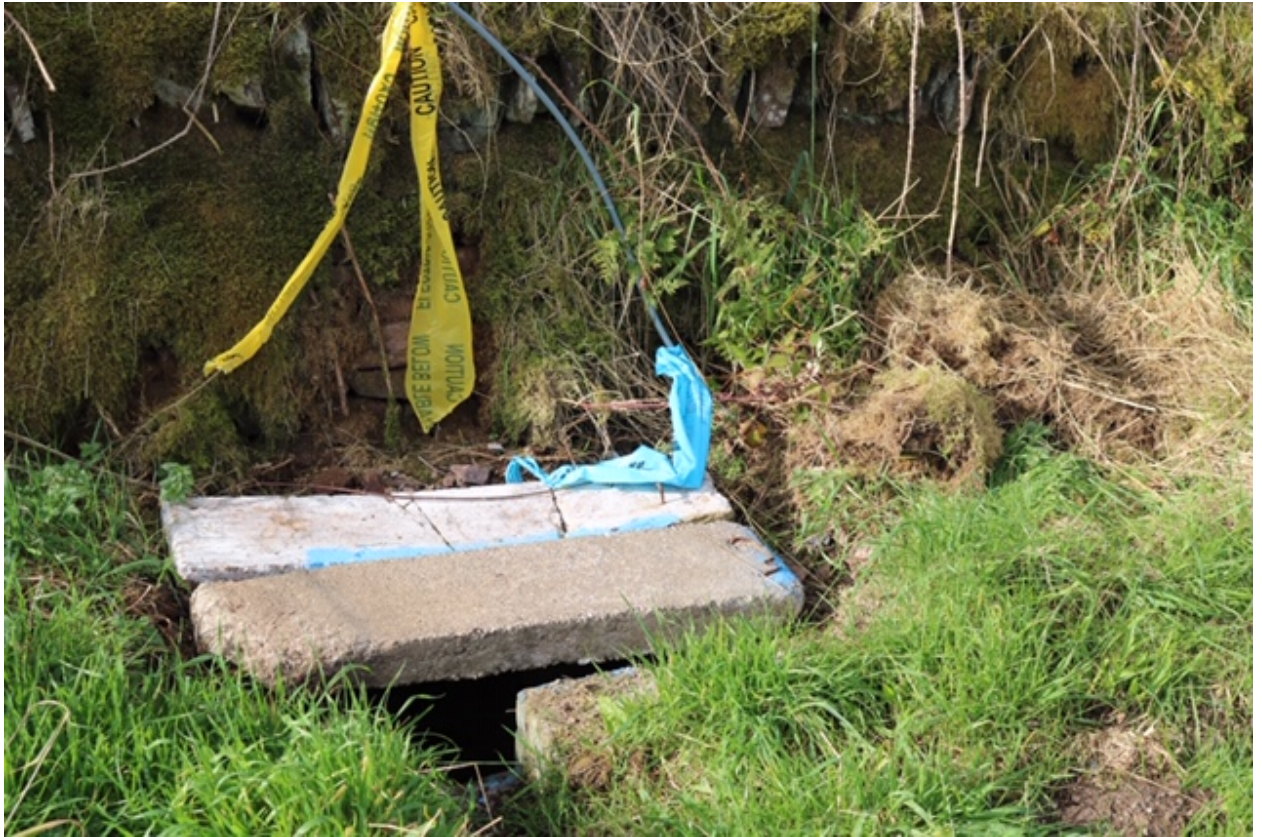
Hidden obstacles within the ditch close to the proposed site entrance
