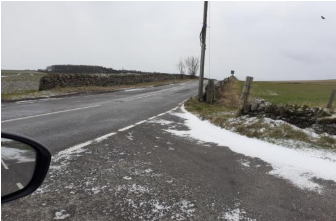
G looking to F At junction with B961, front wheels on the give way lines, looking south on the B961
