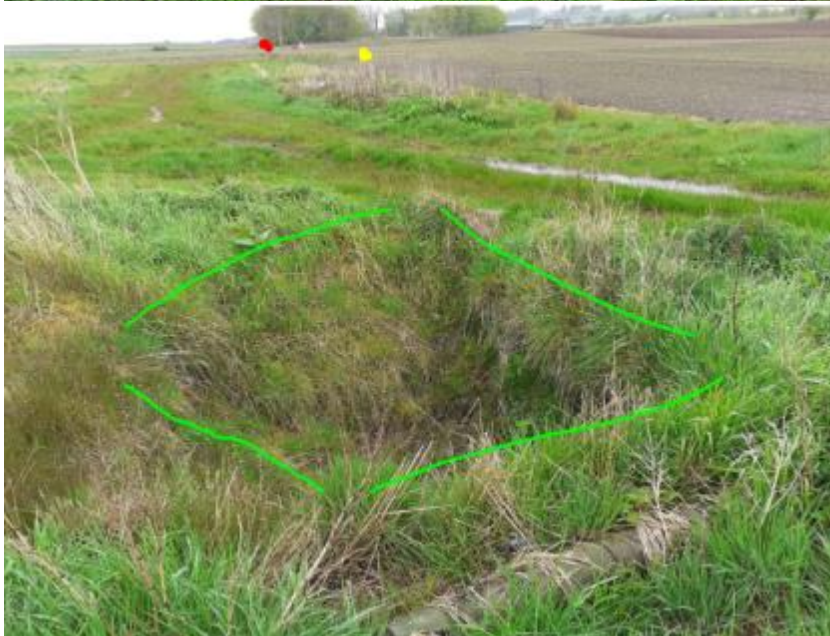
Middle image: showing the positions of, in red, the large active well / cistern, in yellow, the above water pipes, and in green another large square cistern, but this one is redundant, with overgrown sides and a large boulder in the bottom, presumably to cover a hole
