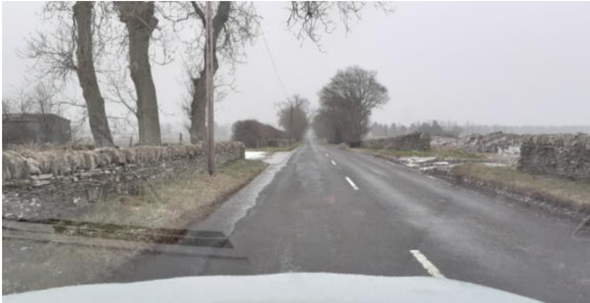
Just south of the opening onto the applicant's land at J Opening is on the left, where the dyke ends
