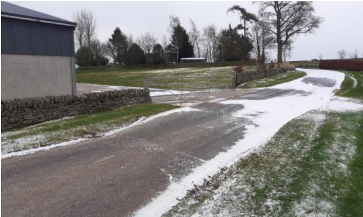
Second existing entrance to applicant's land between D and E, looking towards bend at E
