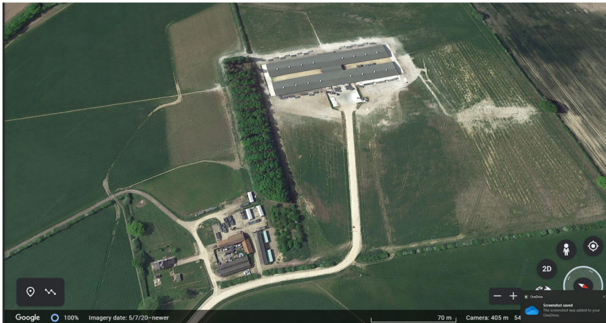
Photo 1 Sally Farm showing two 32k sheds and access road with central staff/ packing facility.
