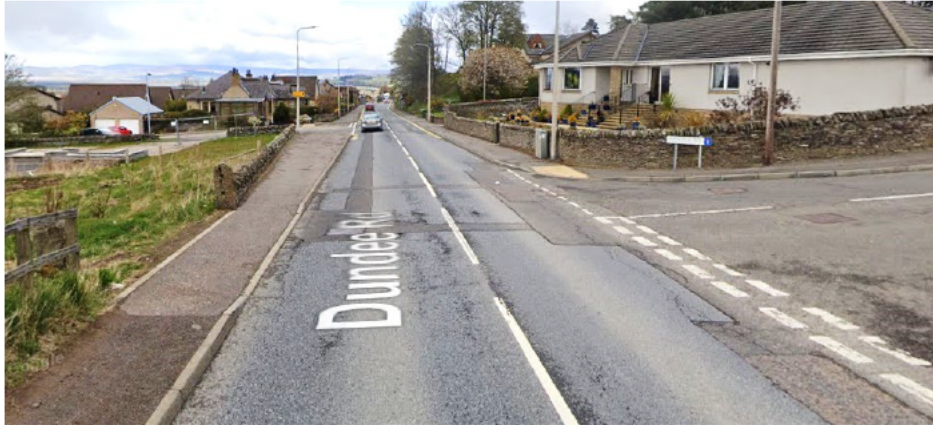
Image 2, footways on Dundee Road (source: Google Streetview)
