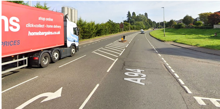
Image 1 , sole existing crossing of Glamis Road (source: Google Streetview)
