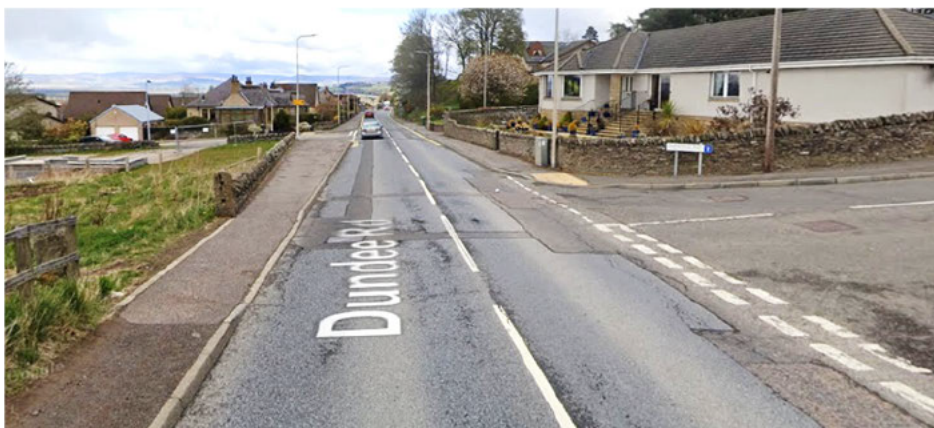
Image 2, footways on Dundee Road (source: Google Streetview)
