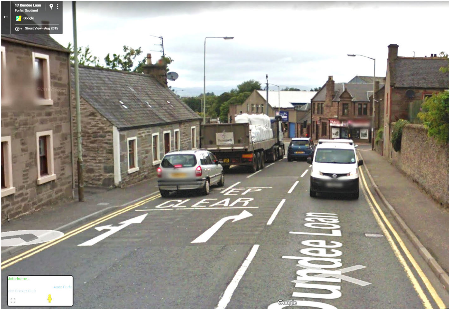
Diagram 22123/2 – A926 Dundee Loan approach to A90 /A926 signals (Source: Google Streetview, not for publication)
