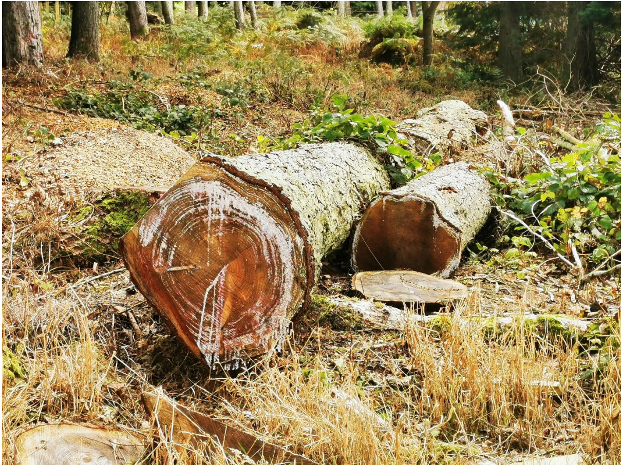
Photo 7 – Trees recently felled and woodland cleared to create proposed driveway
