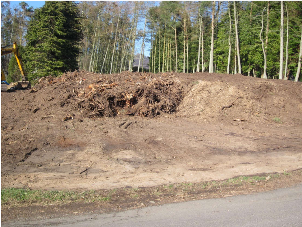
Photo 5 – Woodland at The Whins being cleared. Boundary fence removed.
