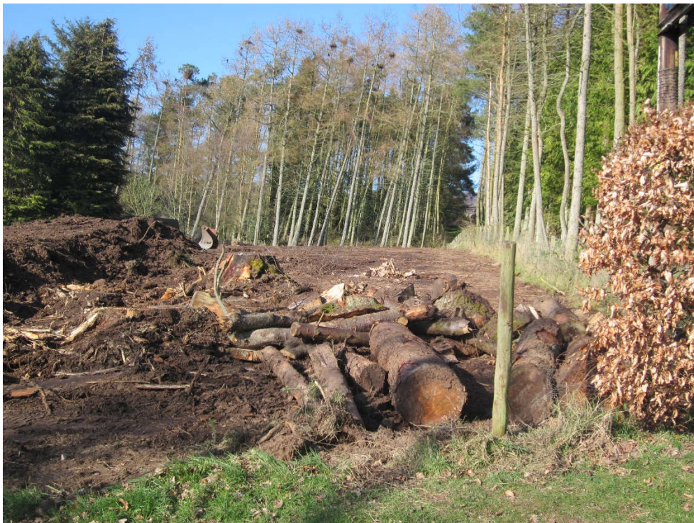
Photo 2 – trees being felled at The Whins to remove woodland.
