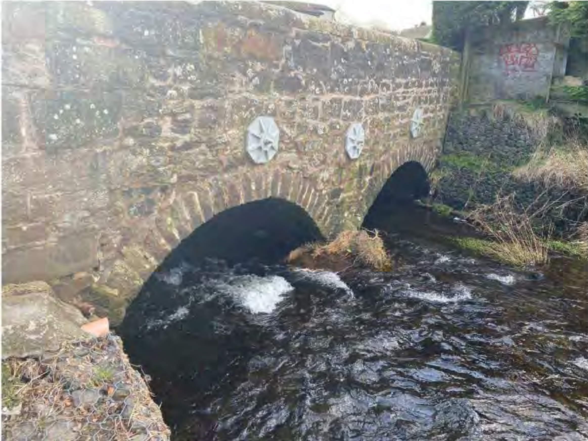
Photograph 5 – upstream side of the Baldovan Road masonry arch bridge.
