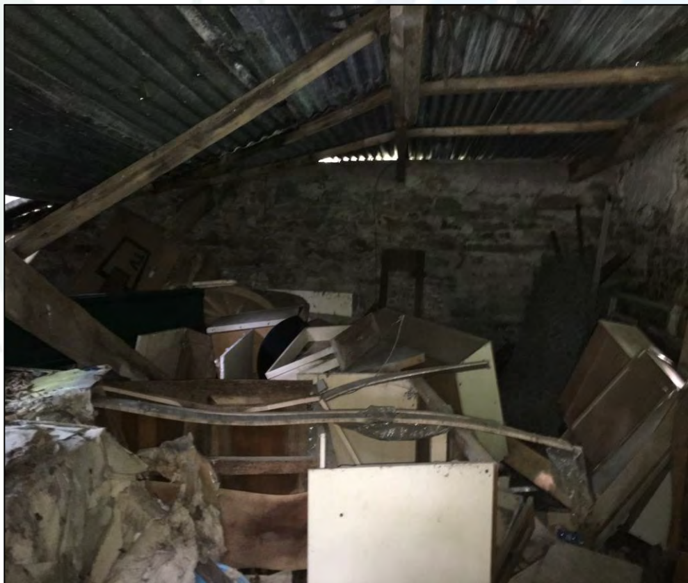
Figure 4. Corrugated sheeting onto wooden joists
