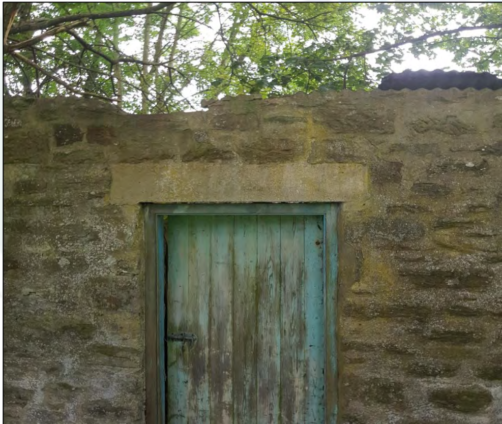
Figure 2. Front of building with stonework in good condition.
