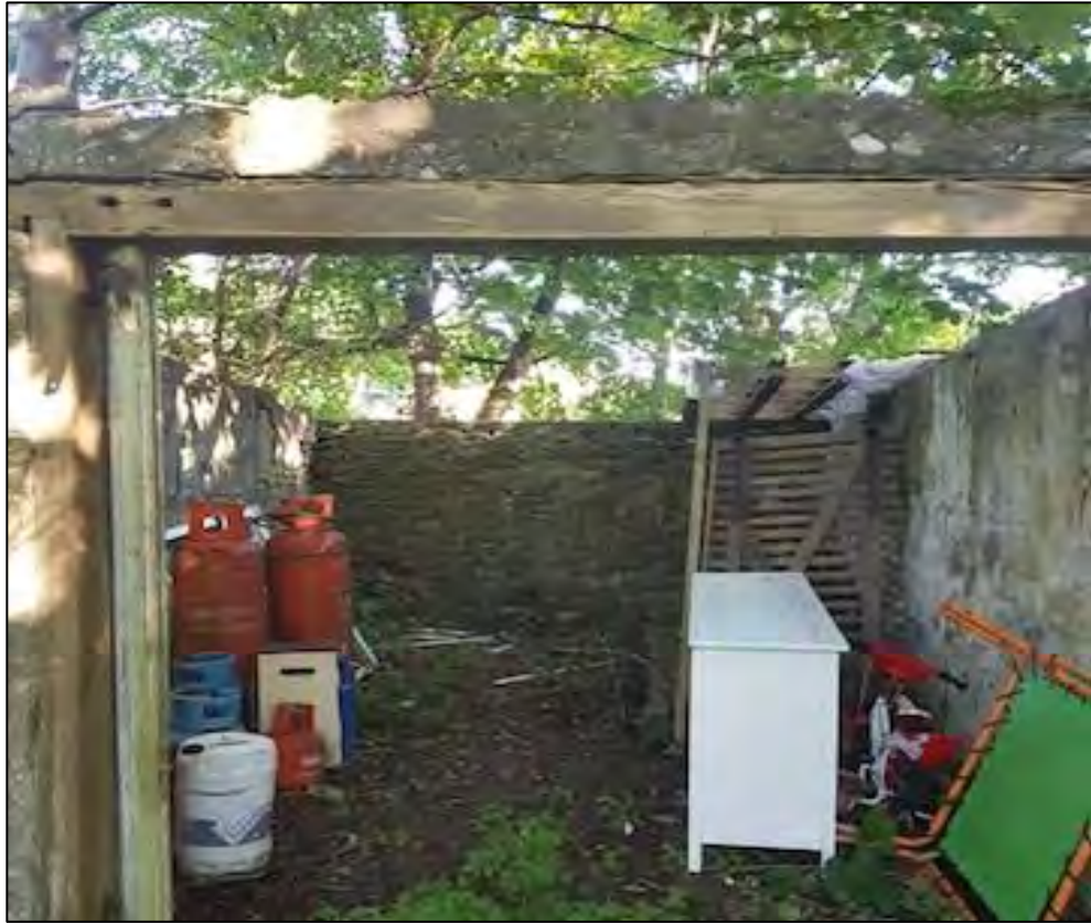
Figure 3. Shell of building with no roof present
