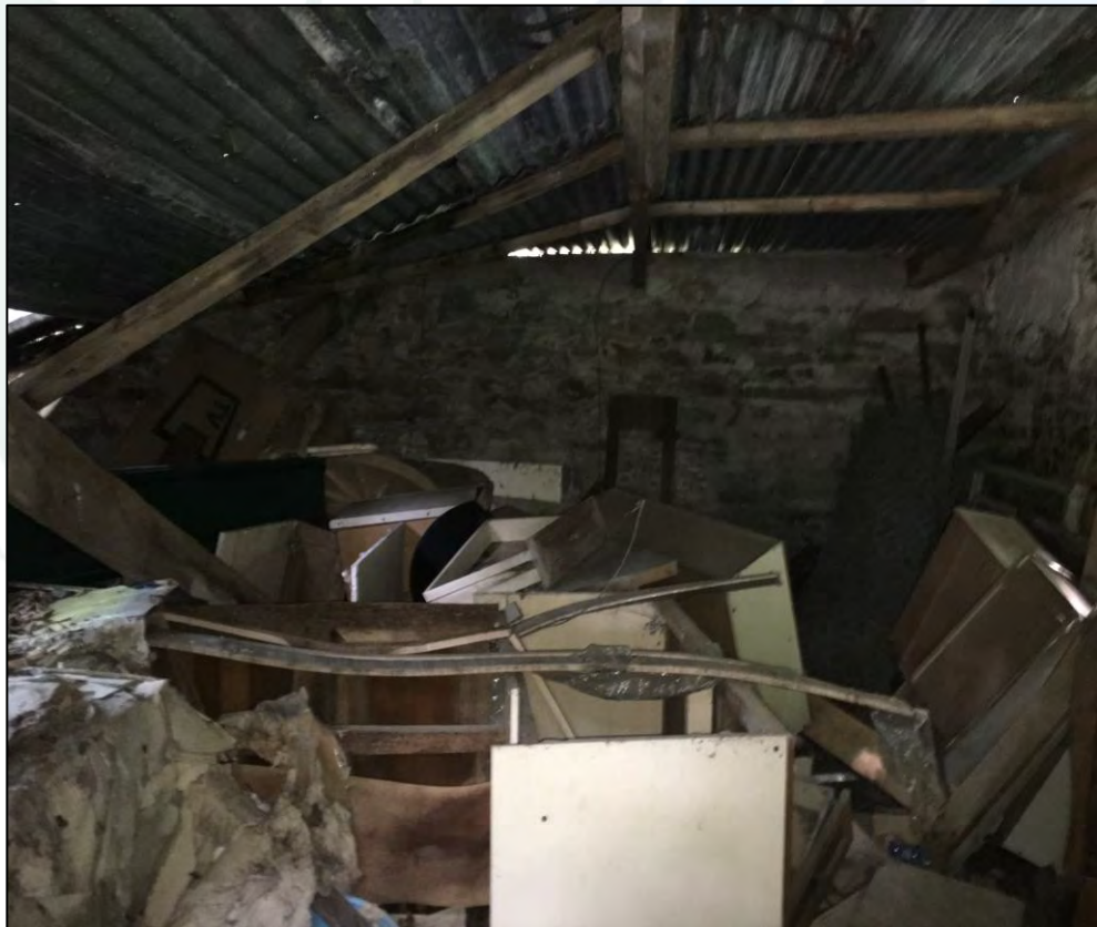
Figure 4. Corrugated sheeting onto wooden joists
