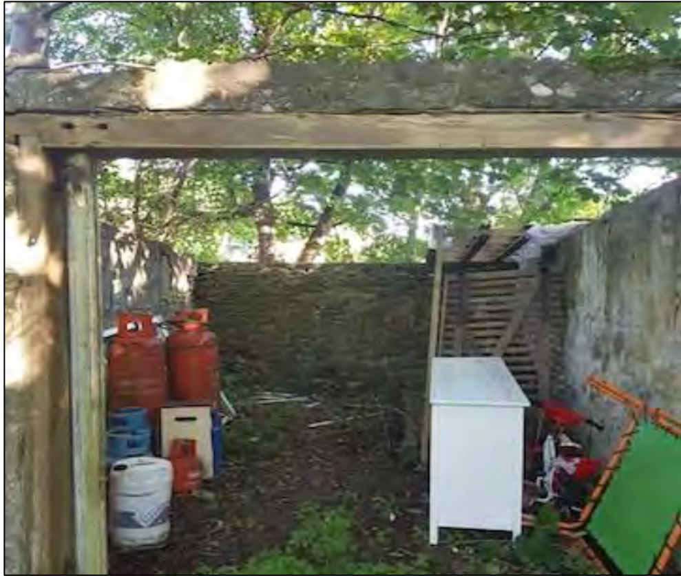
Figure 3. Shell of building with no roof present
