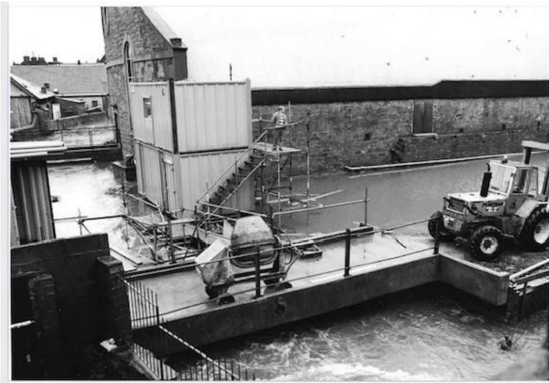
PHOTO B – 1994 extreme flood. Taken from window of Flat at 39 East Grimsby. Water level approx 3.600m.
