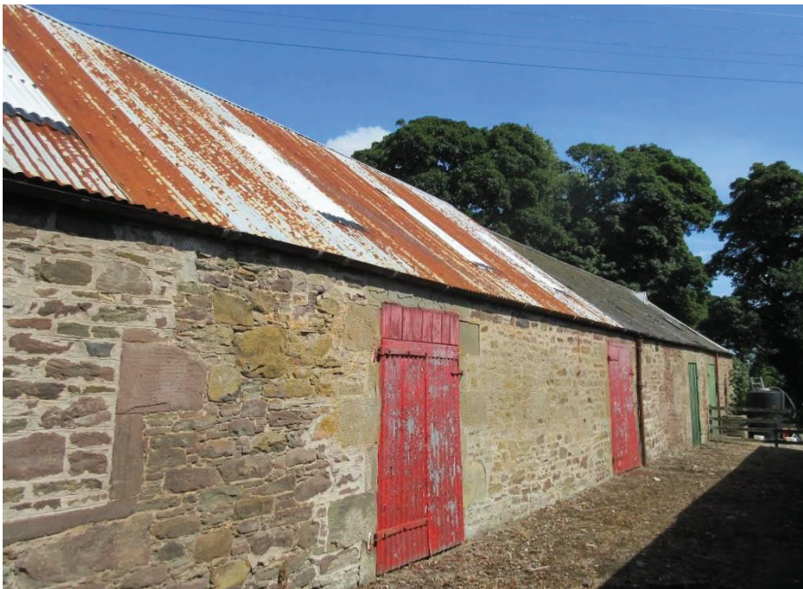
Photo 16. Building N, southern side; part corrugated metal roof, part slate roof.
