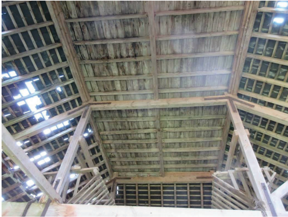
Photo 9. Building G internal.
