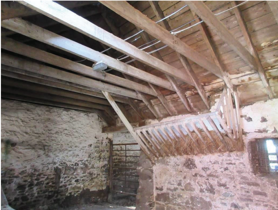
Photo 15. Building M, internal. Gate on right leads into building L.
