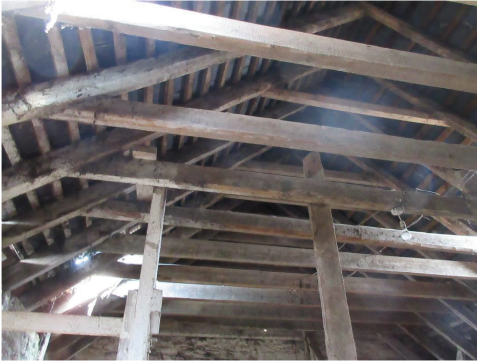
Photo 11. Building I internal.
