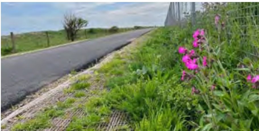
Photo: NCN1Elliot Links path upgrade © Russell Cramb
