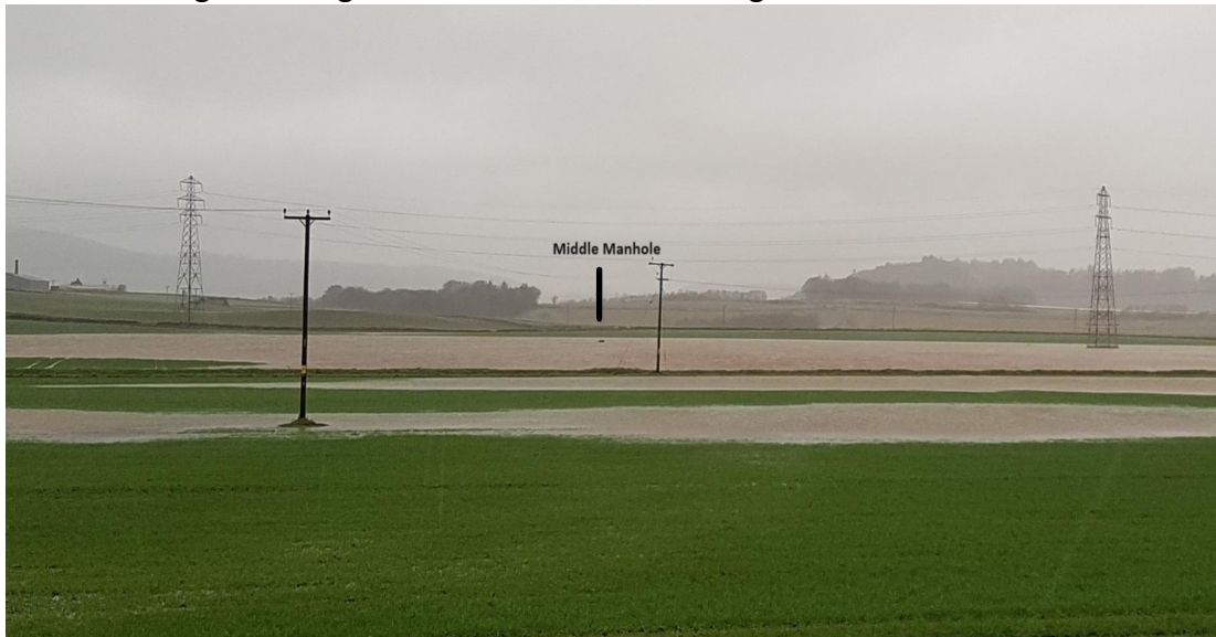
Northern range flooding 18 November 2022 showing flood around middle manhole
