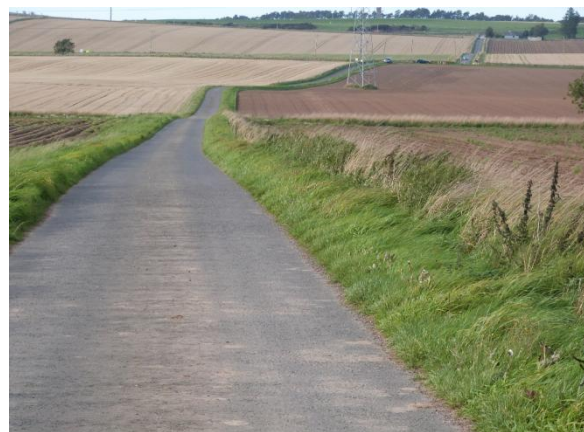
Access road looking north to public road
