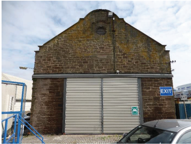
SW elevation (gable)
