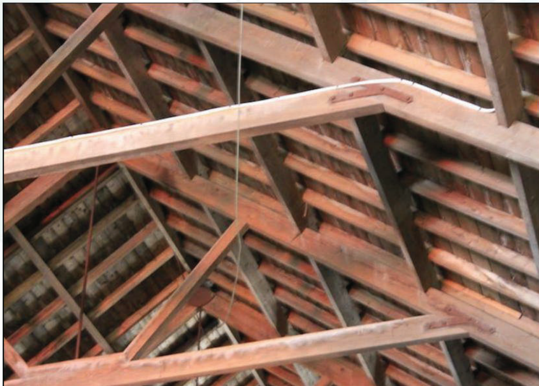
Figure 8. Slates laid onto wooden sarking and joists.
