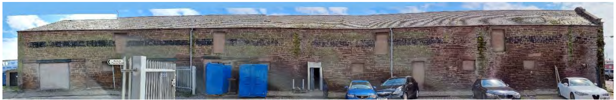
Panoramic image of NW elevation assembled from several separate photographs
