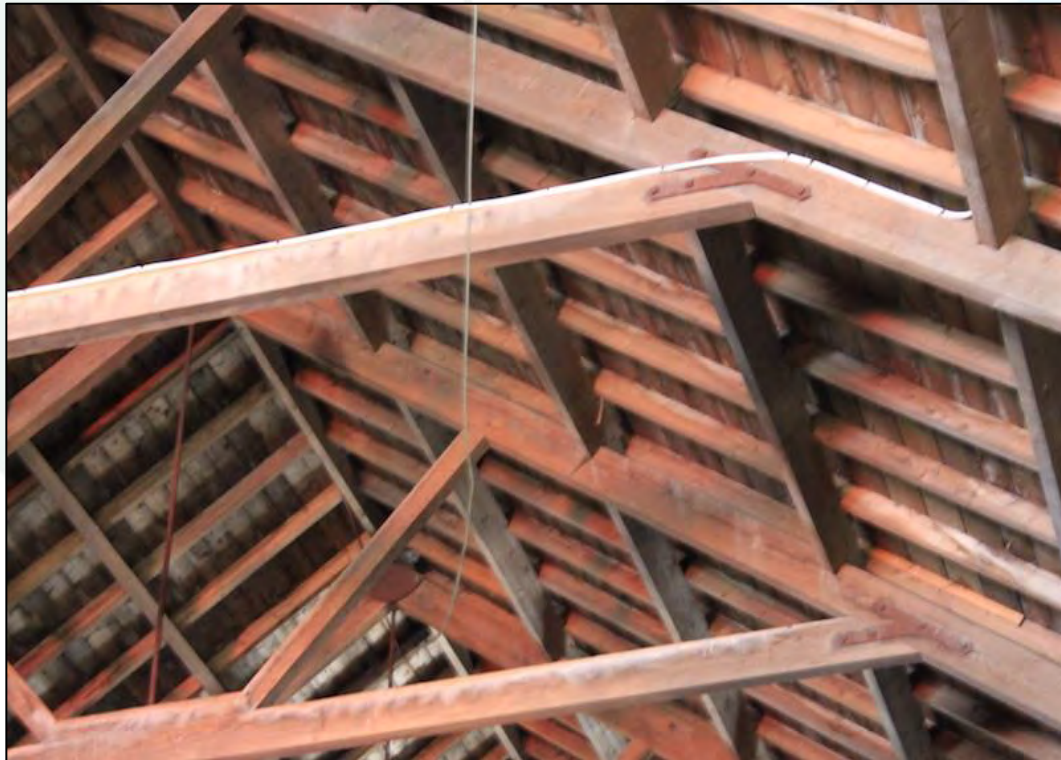
Figure 8. Slates laid onto wooden sarking and joists.
