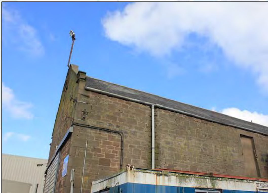
Figure 2. Stonework construction of warehouse.
