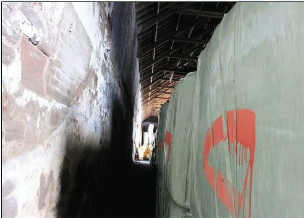
Figure 6. Warehouse actively used for storage.
