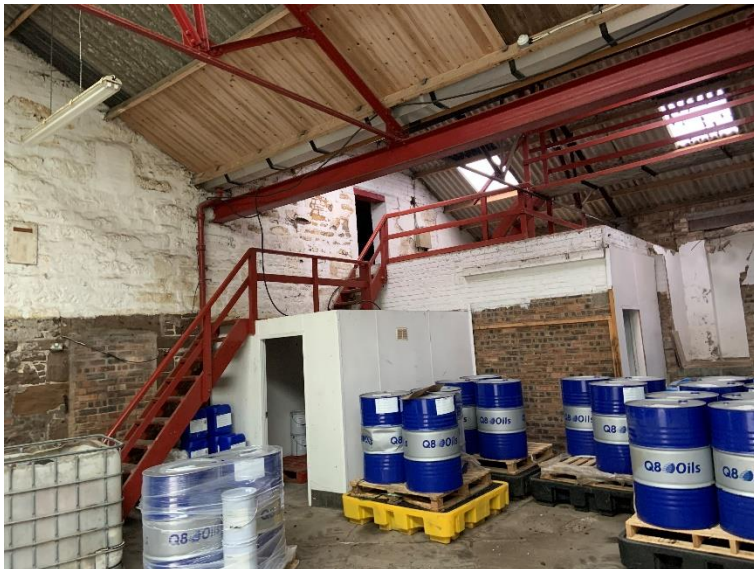
Photograph 4.06 - New Workshop/Store – Internal
