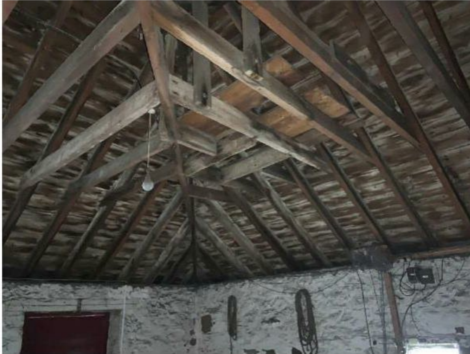
Photograph 3.18 - Old Workshop/Store –America Street Roof
