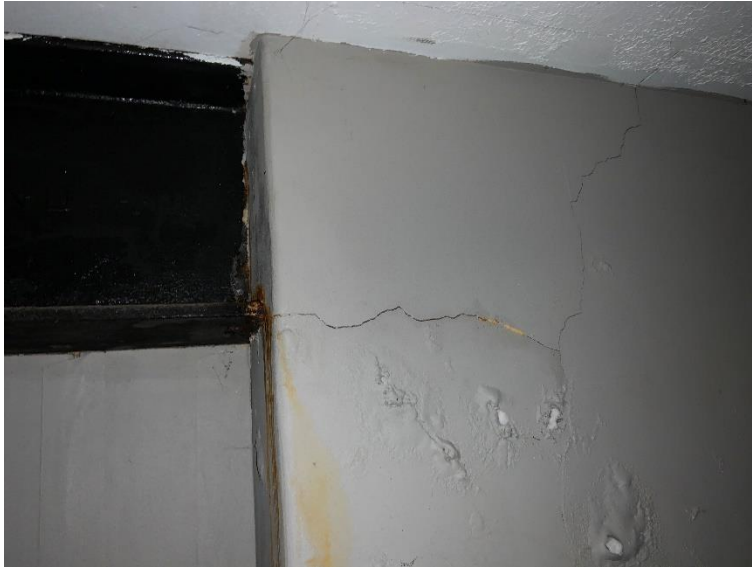
Photograph 3.10 - Old Workshop/Store – Steel Beams Support
