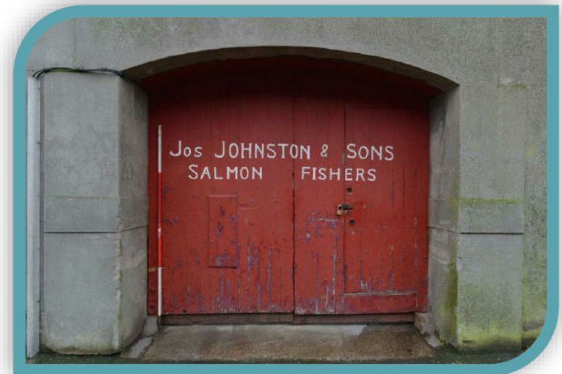
Figure 11: Arched entrance – America Street
