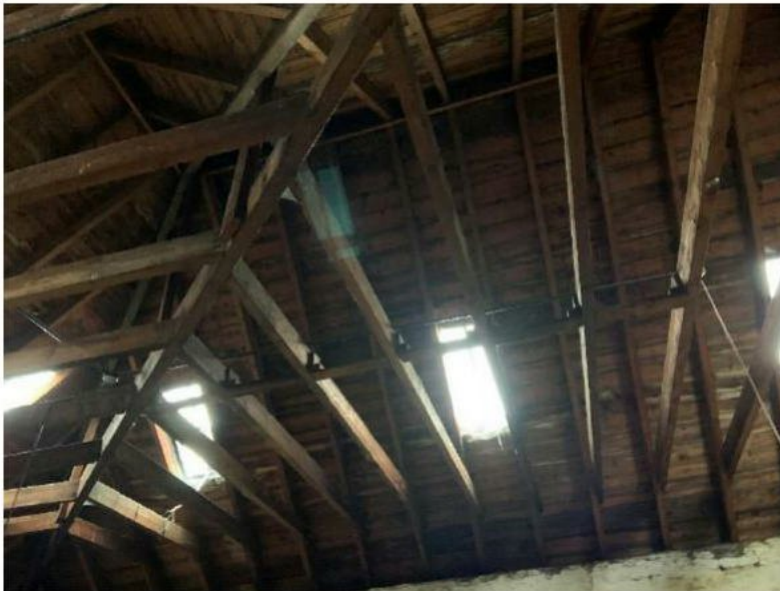
Photograph 3.19 - Old Workshop/Store –California Street Roof
