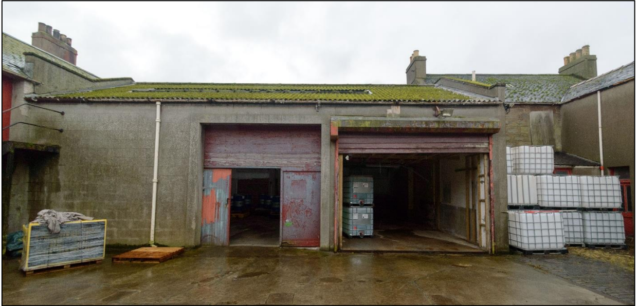
Illus 14 The SW courtyard elevation comprising the substantial garage or warehouse extension (room 10).
