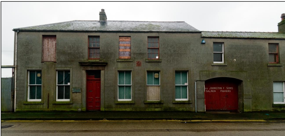
Illus 6 Nos 3 & 4, America Street, façade.
