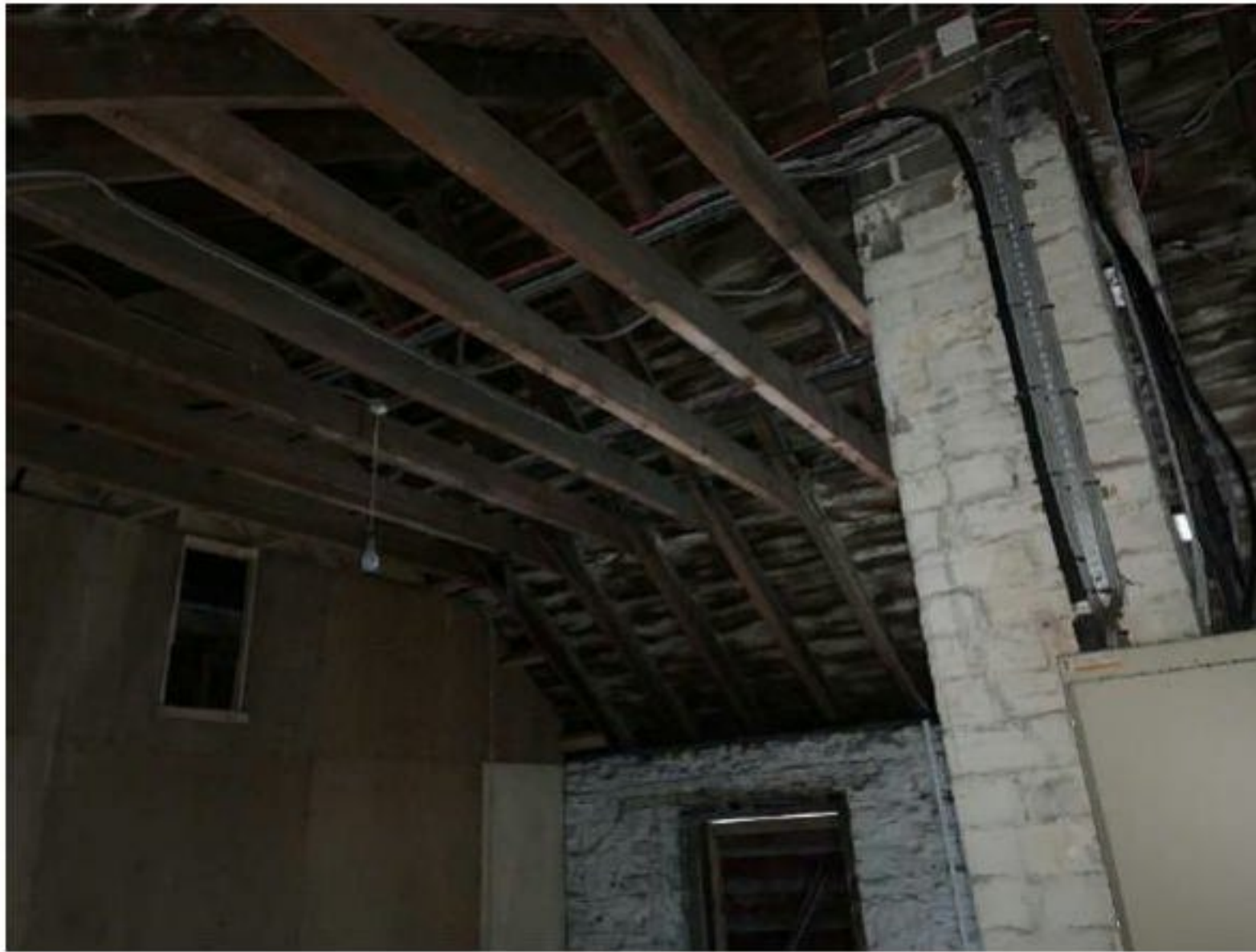
Photograph 3.14 - Old Workshop/Store – Upper Floor America Street
