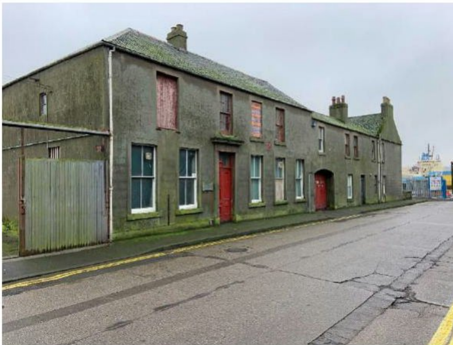
Photograph 2.01 America Street Offices - External Elevation
