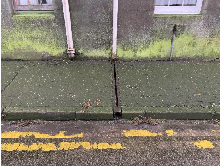
Photograph 1.04 Managers House - External Wall – Gable Drain
