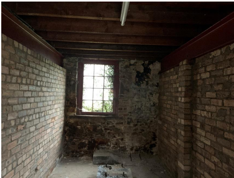
Photograph 3.11 - Old Workshop/Store – Steel Beams / Brick Walls / Floor Joists
