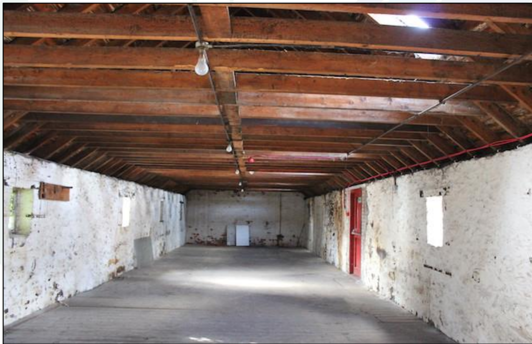
Figure 11. Interior detail with no ceiling or roof cavities present.
