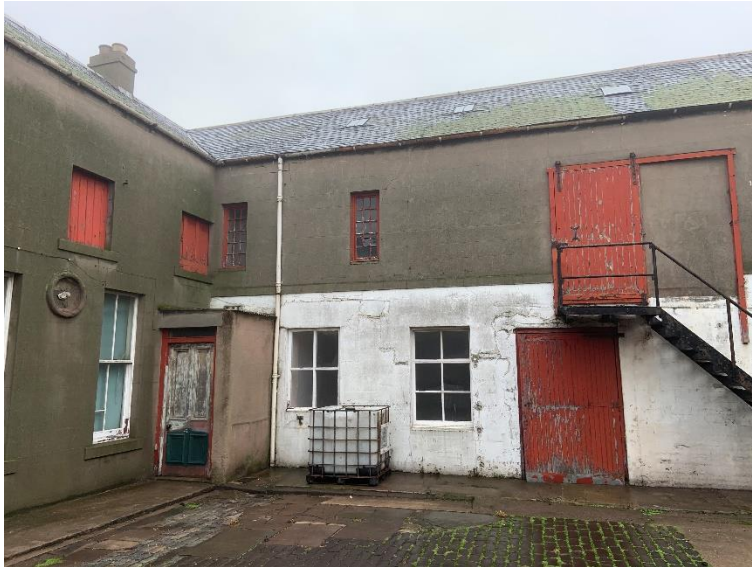
Photograph 3.04 - Old Workshop/Store – Quadrangle Elevation 1
