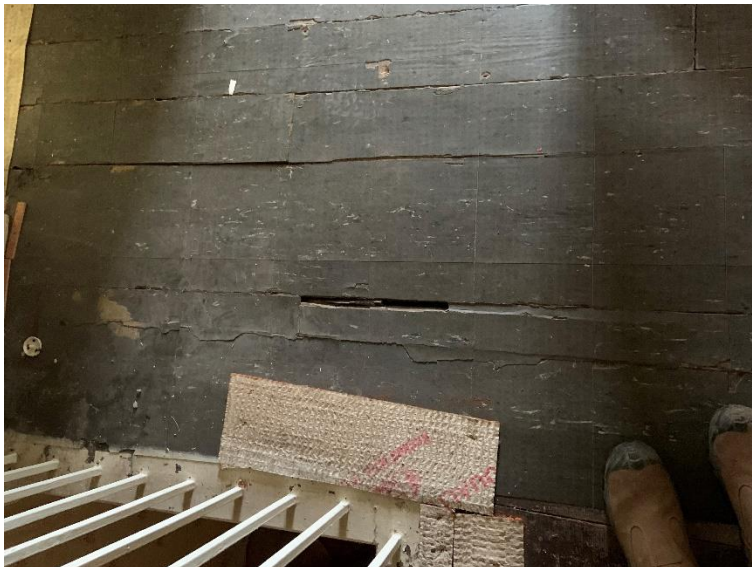
Photograph 1.07 Managers House – 1 st Floor
