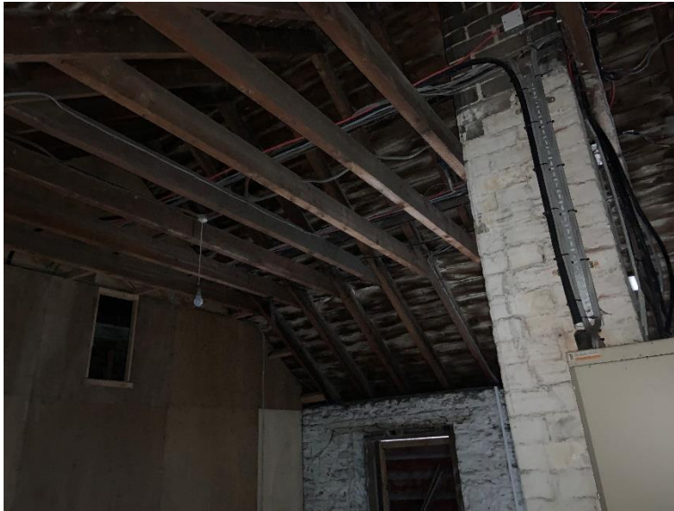
Photograph 3.14 - Old Workshop/Store – Upper Floor America Street
