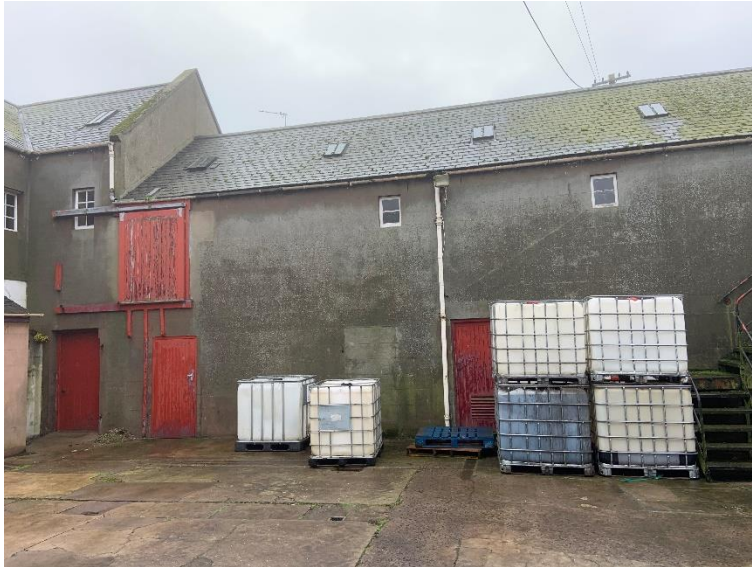
Photograph 3.06 - Old Workshop/Store – Quadrangle Elevation 2
