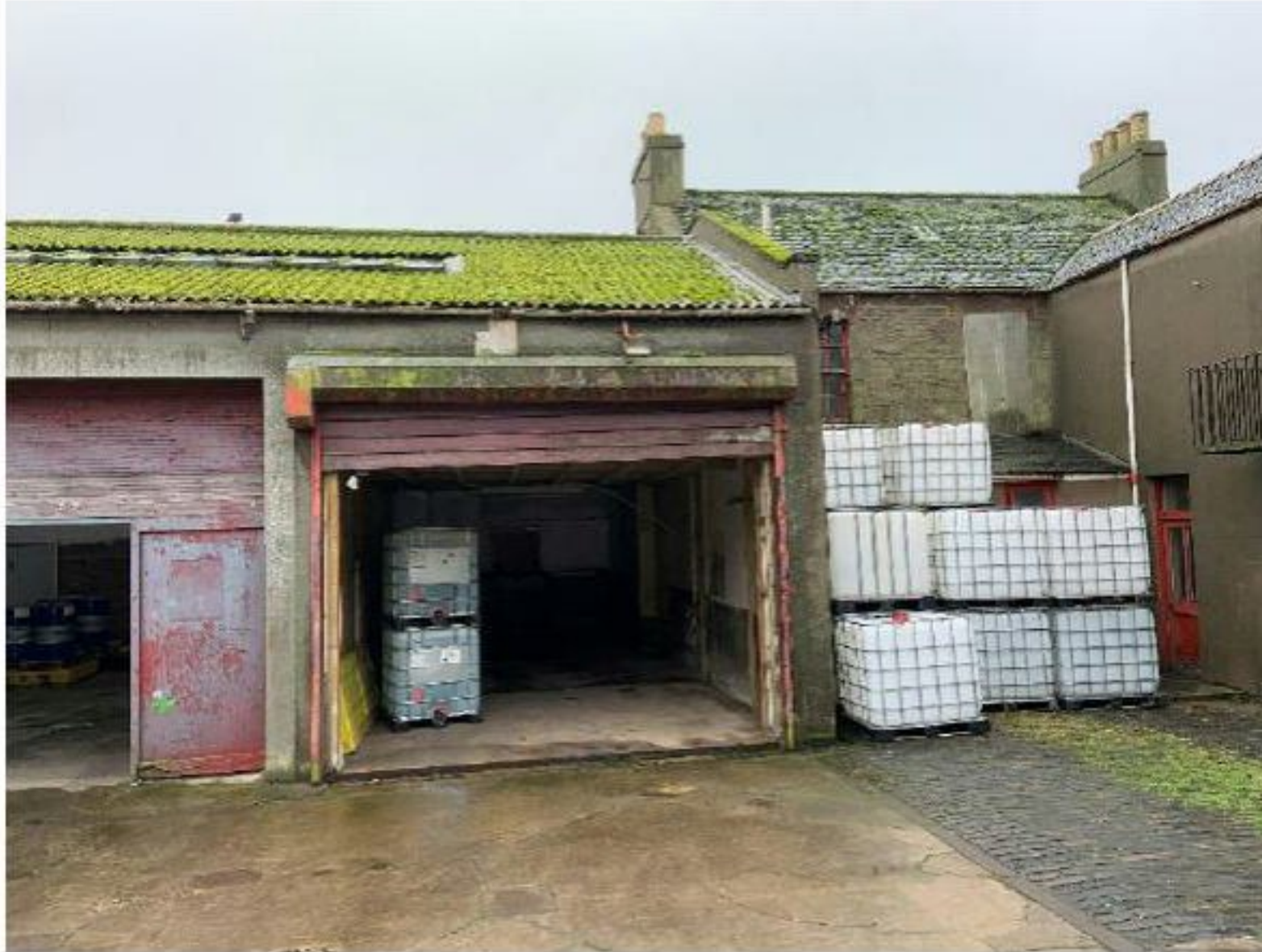
Photograph 1.06 Managers House - External Wall – Rear Elevation
