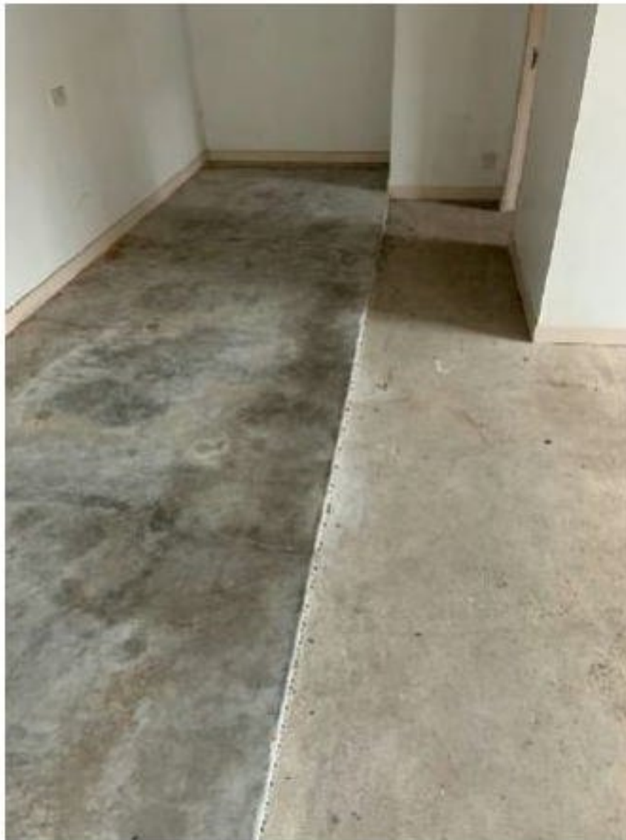
Photograph 3.07 - Old Workshop/Store – Ground Floor
