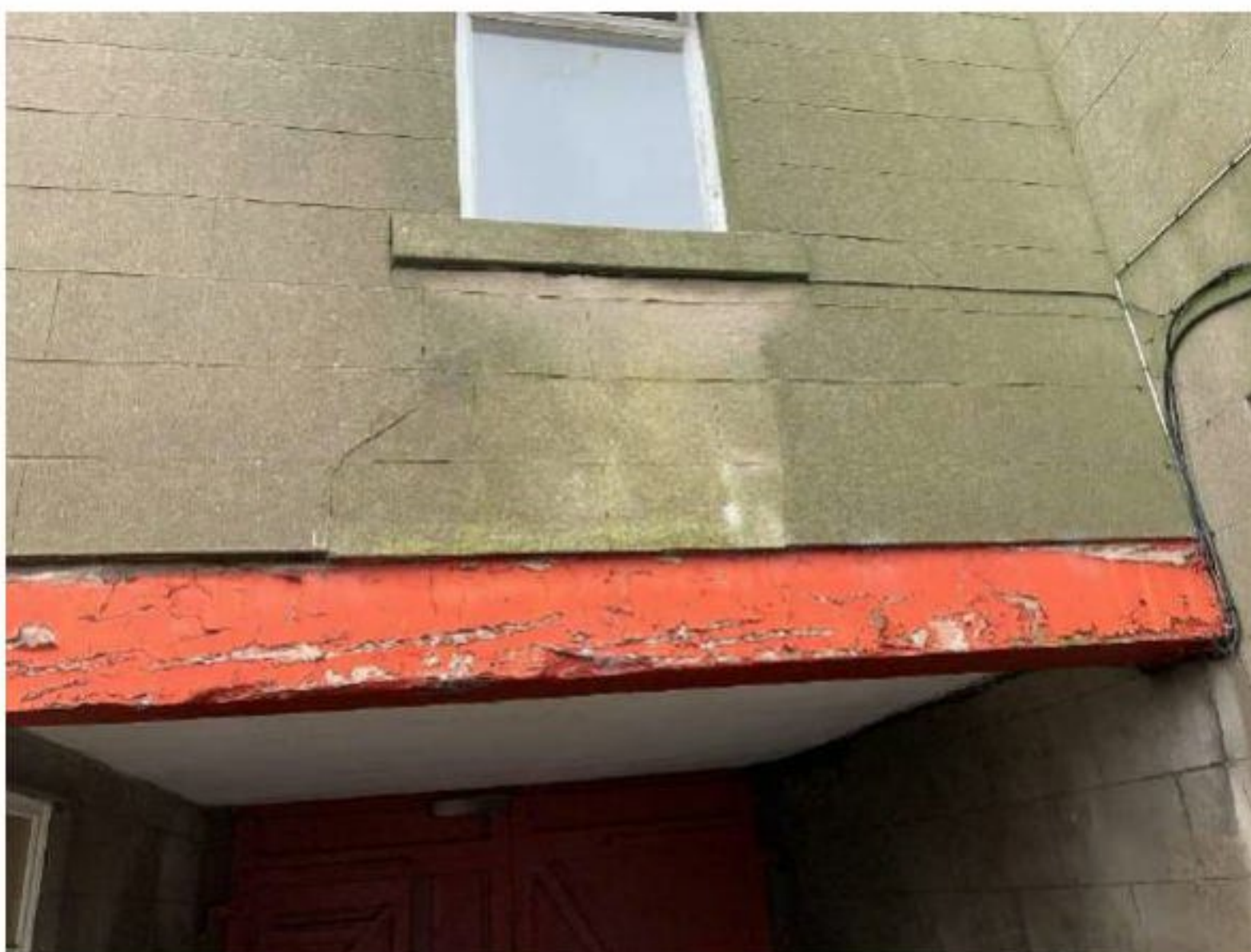
Photograph 2.07 America Street Offices - Quadrangle External Elevation – Arch Lintel
