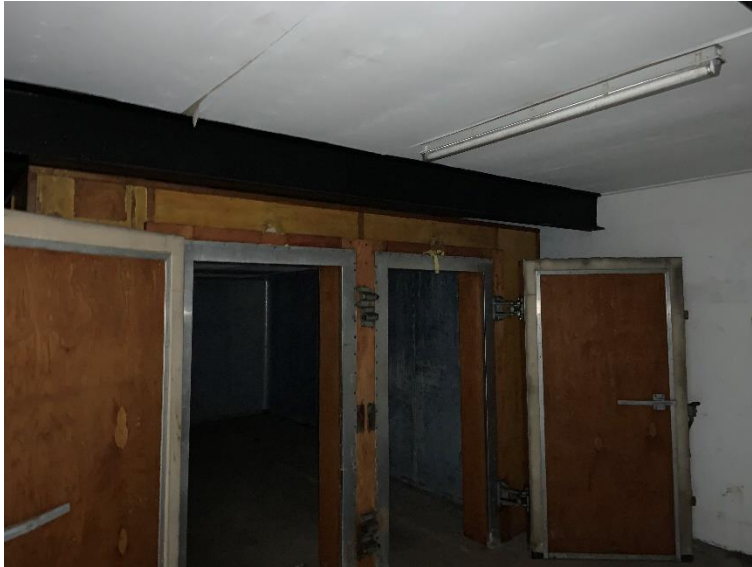
Photograph 3.12 - Old Workshop/Store – Specialist Room 1
