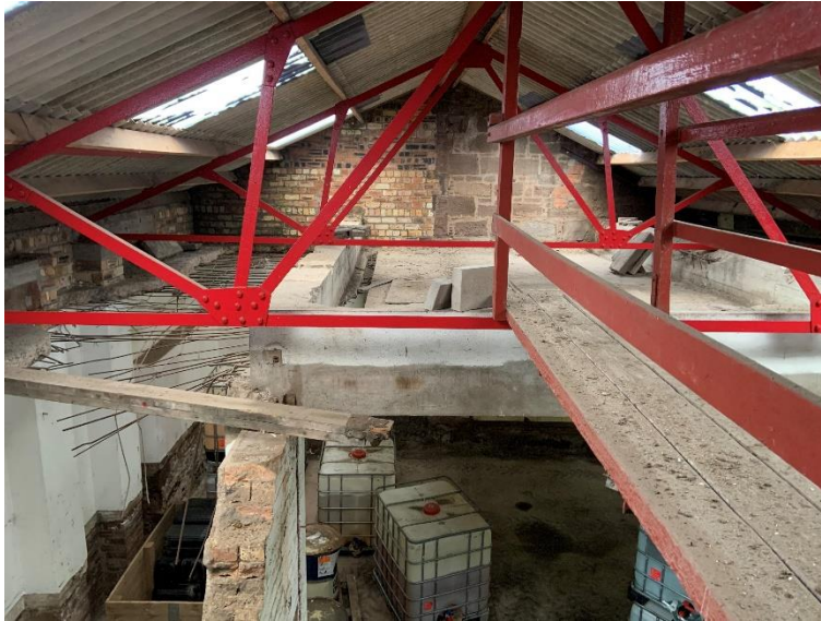
Photograph 4.02 - New Workshop/Store - Roof
