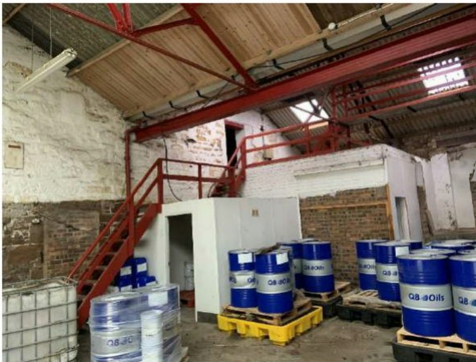
Photograph 4.06 - New Workshop/Store – Internal
