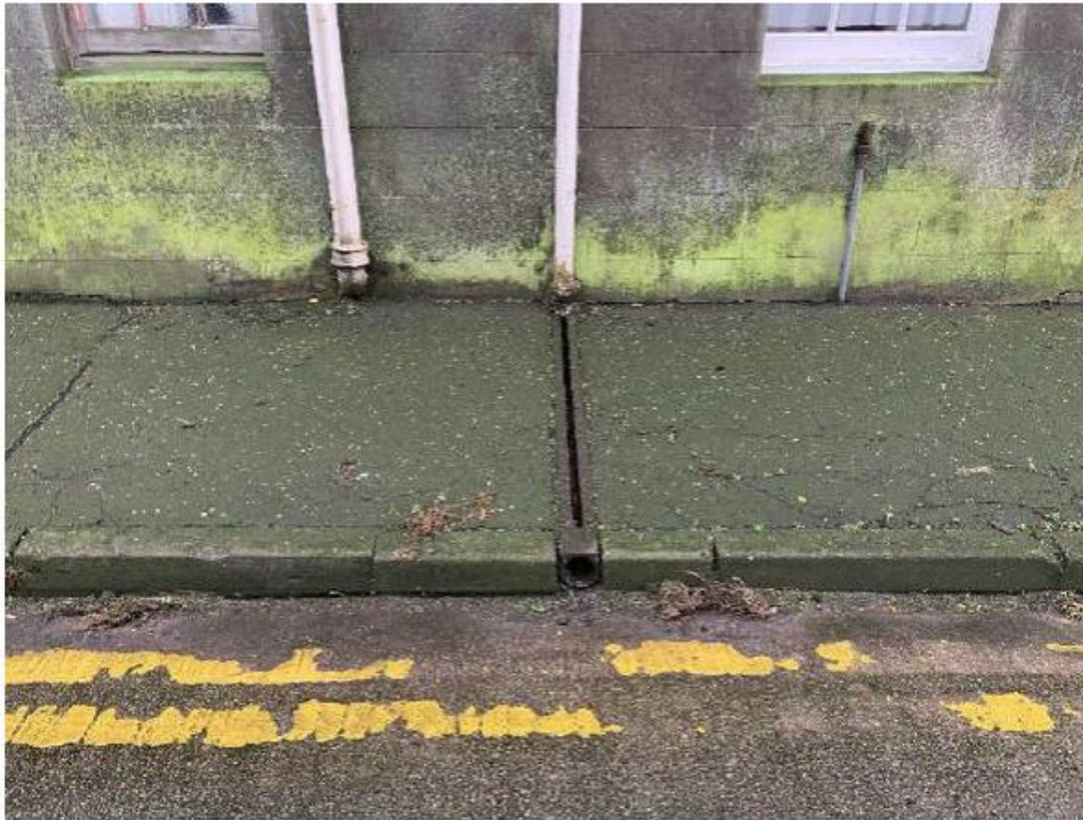
Photograph 1.04 Managers House - External Wall – Gable Drain
