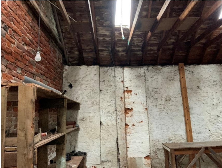
Photograph 3.16 - Old Workshop/Store – Upper Floor Central Section / California Street Corner
