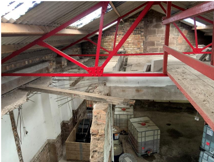
Photograph 4.08 - New Workshop/Store – Reinforced Concrete/Floor
