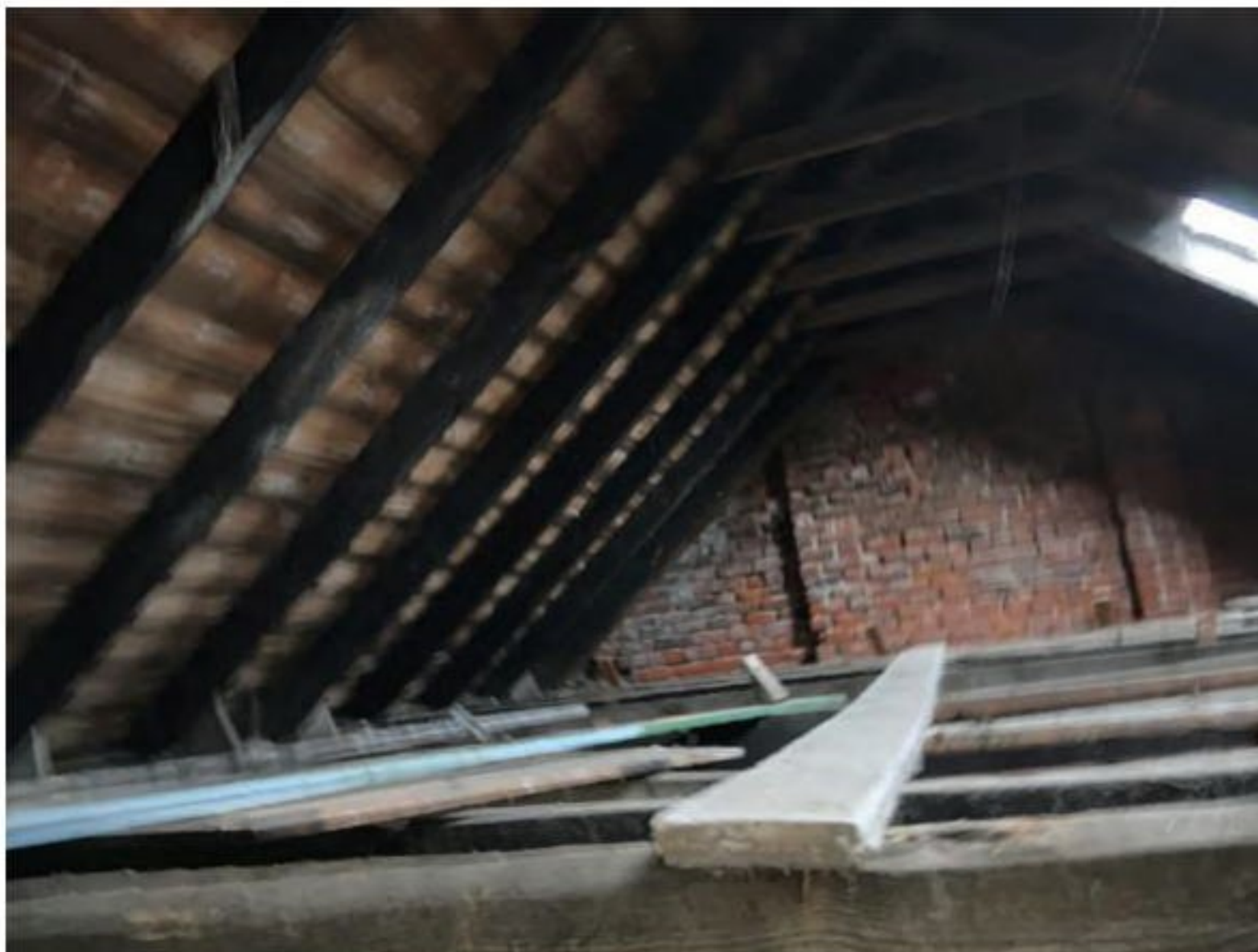
Photograph 3.02 - Old Workshop/Store - Roof
