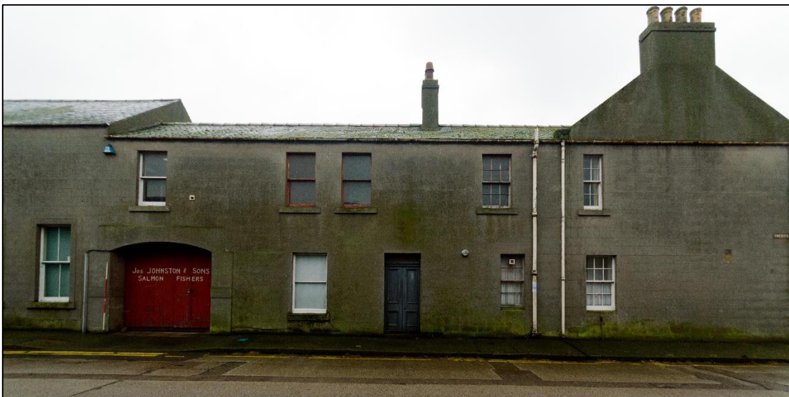
Illus 7 Nos 4 & 5, America Street, façade.
