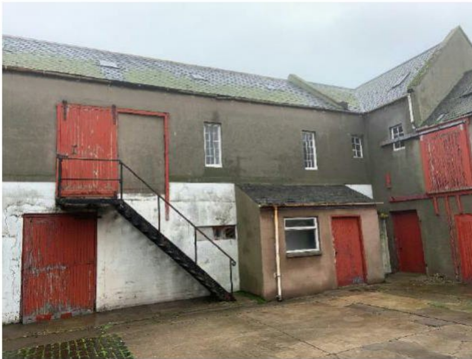
Photograph 3.05 - Old Workshop/Store – Quadrangle Elevation 2
