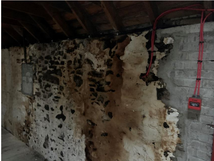
Photograph 3.20 - Old Workshop/Store –California Street Wall
