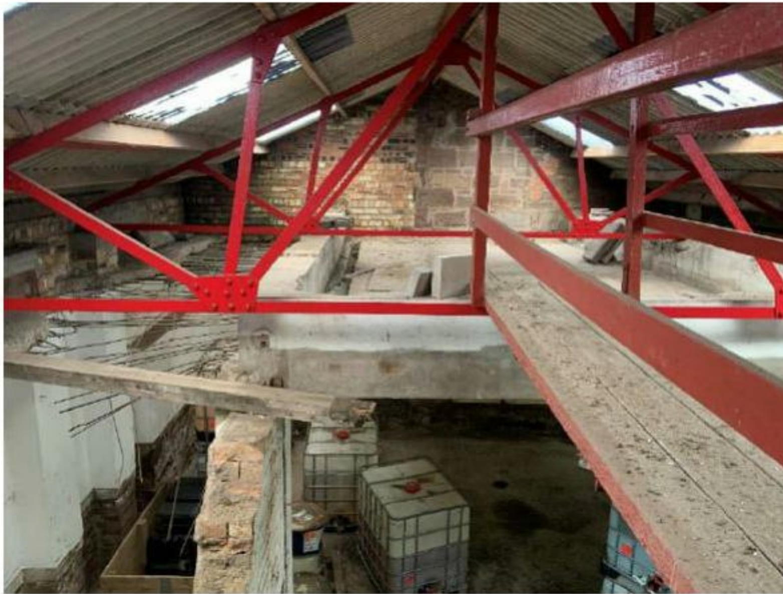
Photograph 4.02 - New Workshop/Store - Roof
