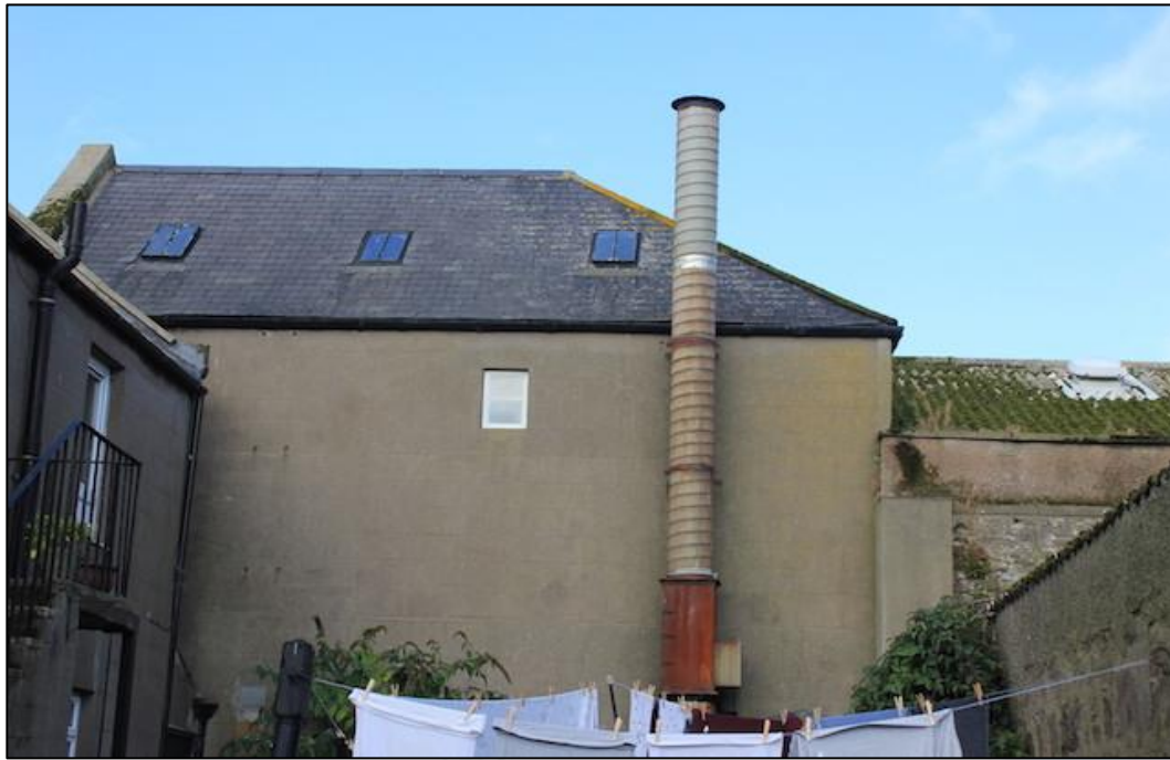
Figure 6. Stonework in good condition.
