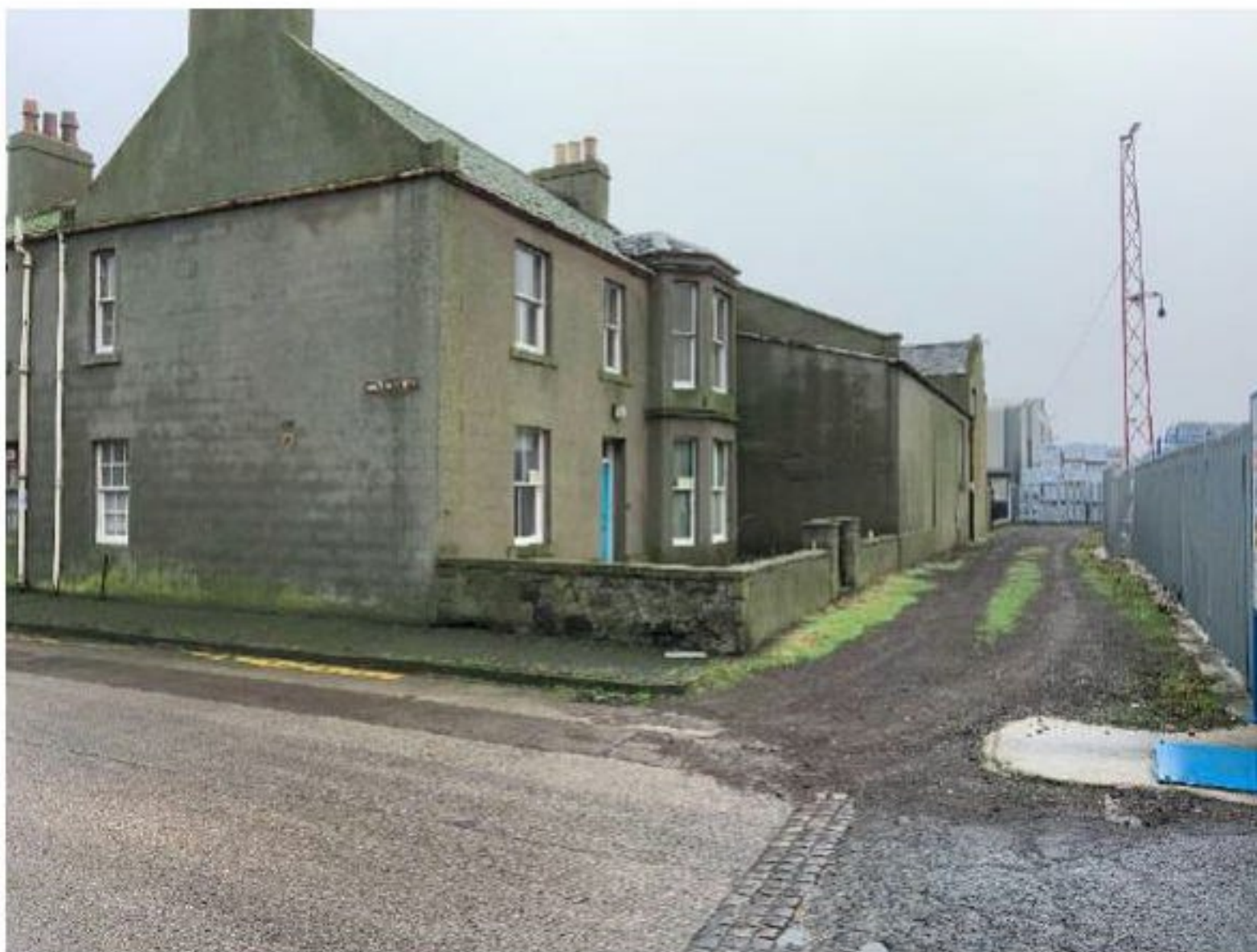
Photograph 1.05 Managers House - External Wall - Gable
