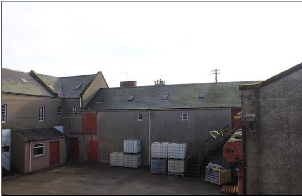
Figure 8. Interior courtyard to be demolished.
