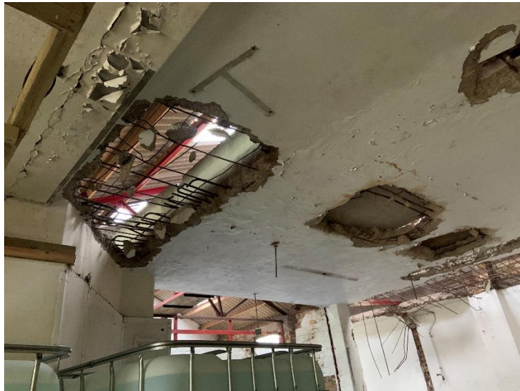
Photograph 4.09 - New Workshop/Store – Reinforced Concrete/Floor
