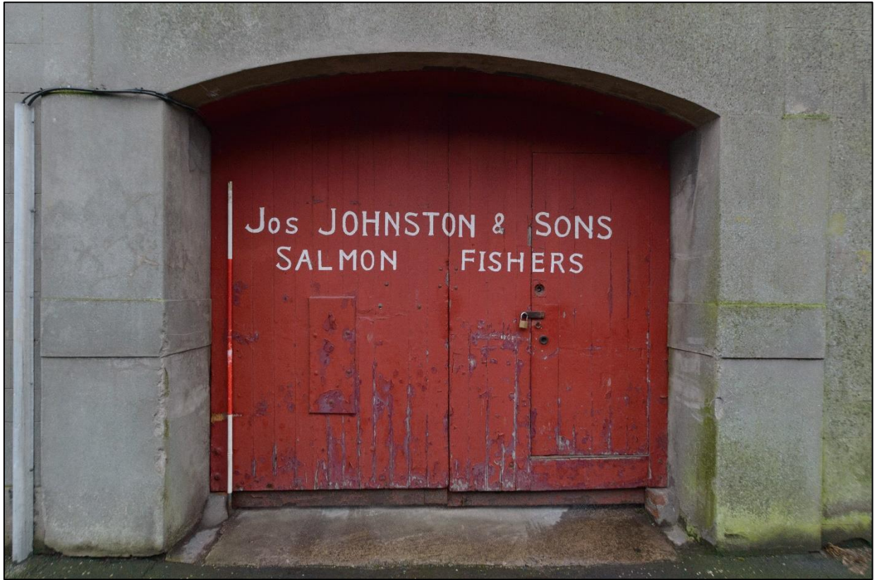
Illus 8 Detail view of D2, main entranceway to courtyard.
