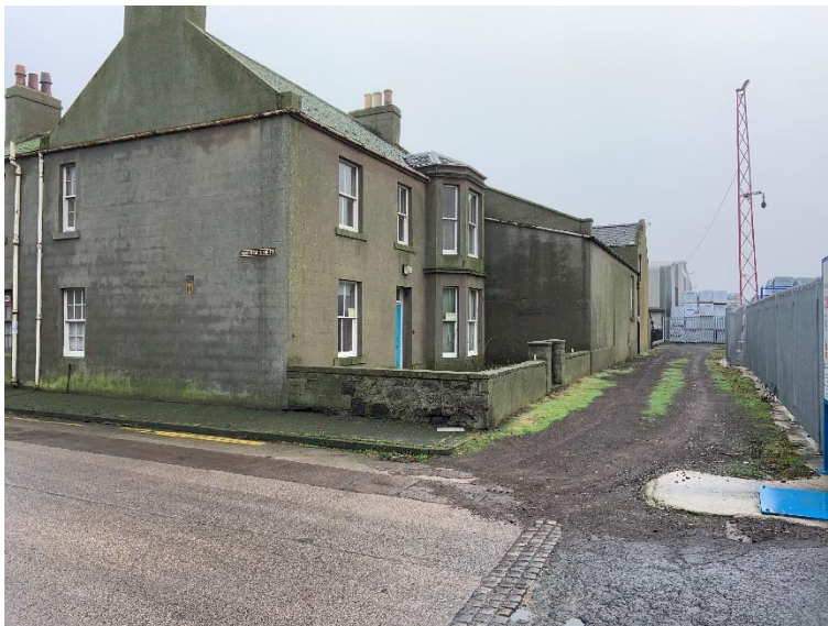
Photograph 1.05 Managers House - External Wall - Gable
