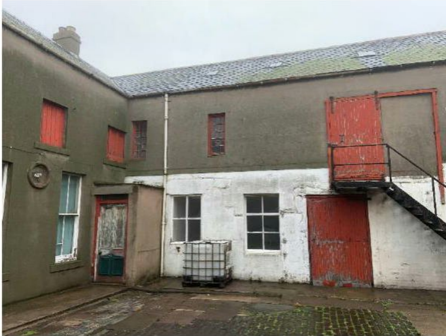
Photograph 3.04 - Old Workshop/Store – Quadrangle Elevation 1
