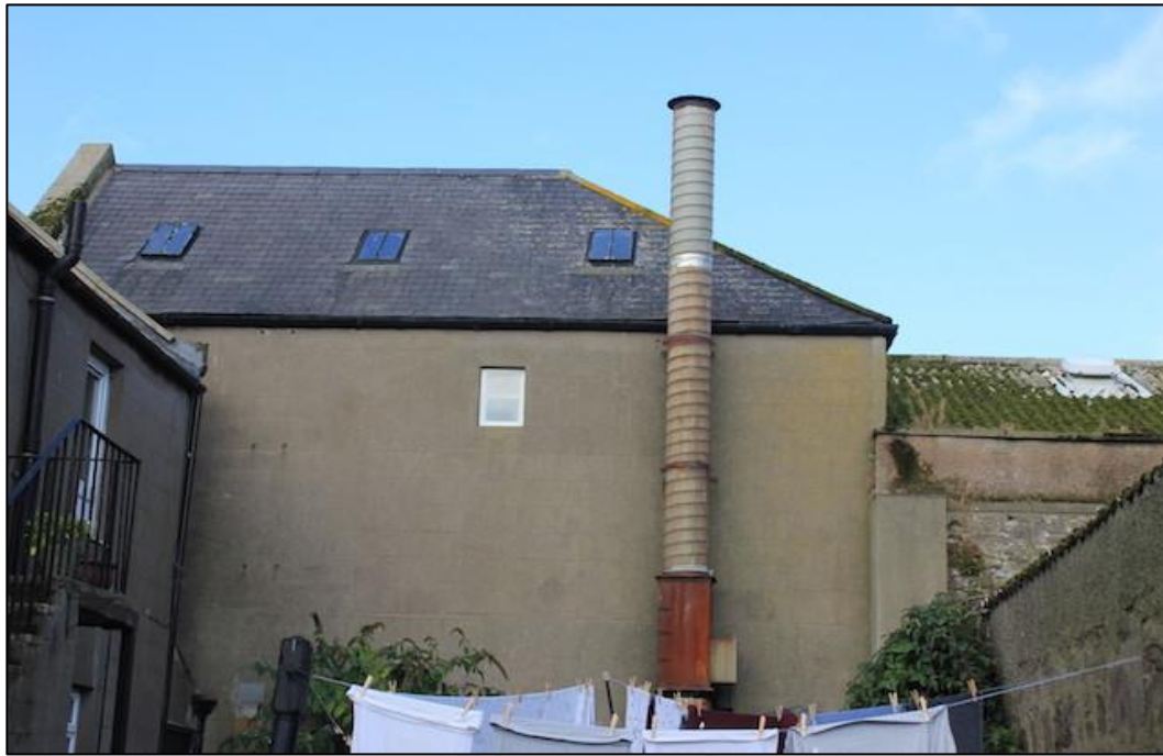
Figure 6. Stonework in good condition with no bat roost potential.
