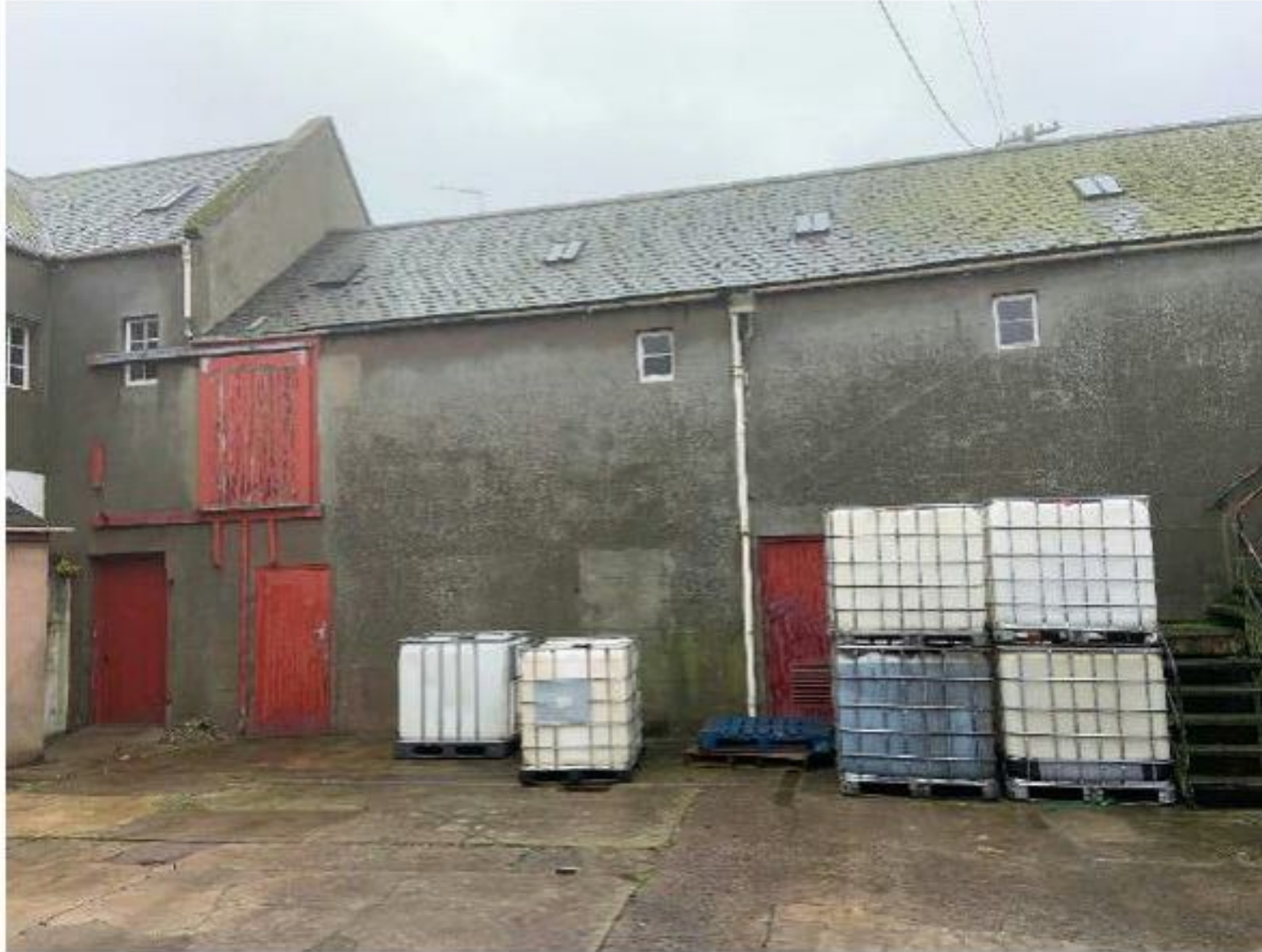
Photograph 3.06 - Old Workshop/Store – Quadrangle Elevation 2
