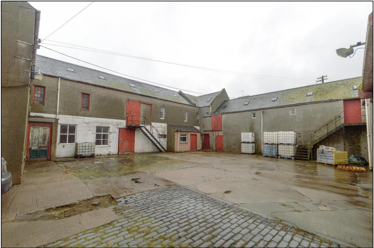
Illus 12 Internal courtyard – general view of SE and NE Elevations.
