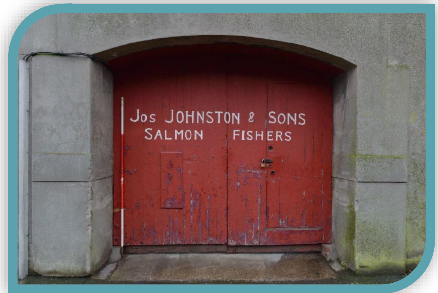
Figure 11: Arched entrance – America Street
