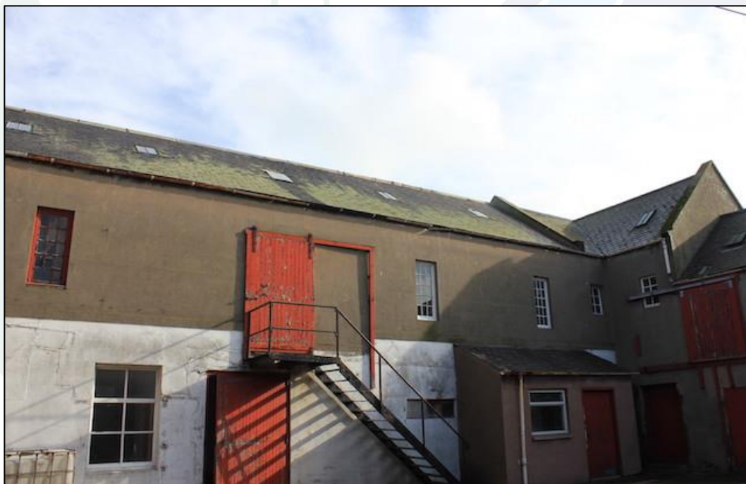
Figure 9. Interior courtyard to be demolished.
