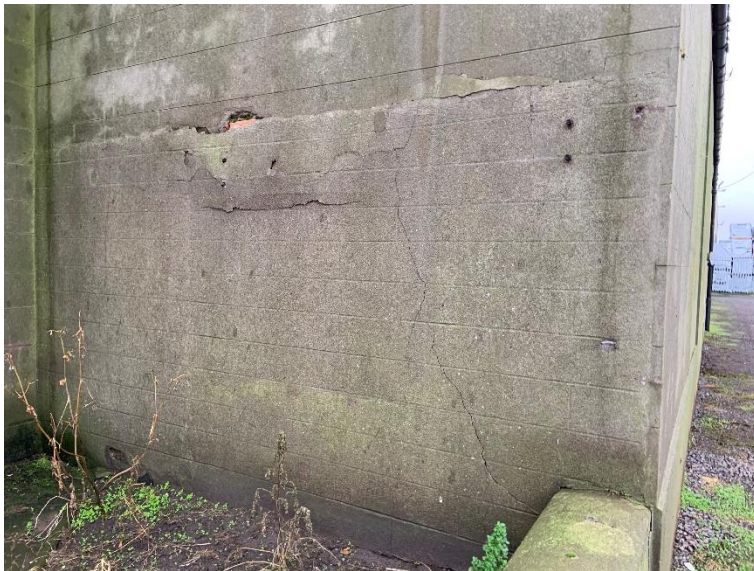
Photograph 4.04 - New Workshop/Store – Return to Managers Office
