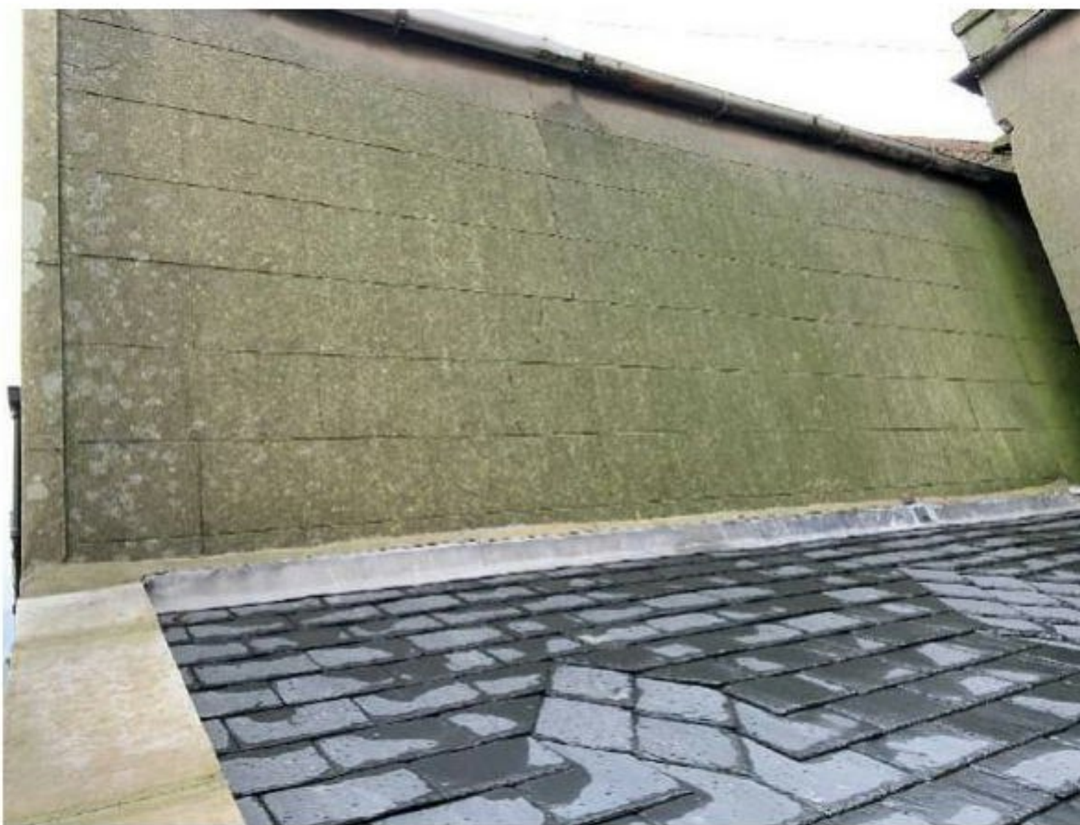
Photograph 3.03 - Old Workshop/Store – California Street Elevation
