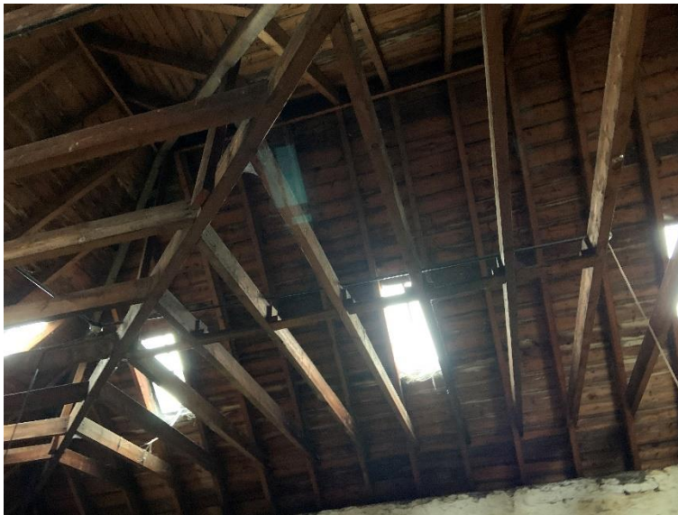
Photograph 3.19 - Old Workshop/Store –California Street Roof
