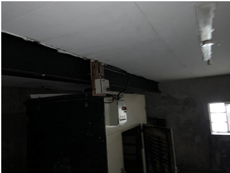
Photograph 3.09 - Old Workshop/Store – Steel Beams
