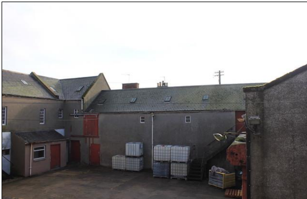
Figure 8. Interior courtyard to be demolished.
