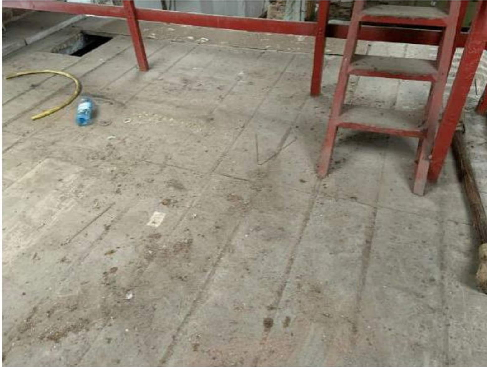
Photograph 4.07 - New Workshop/Store – Precast Ceiling/Floor
