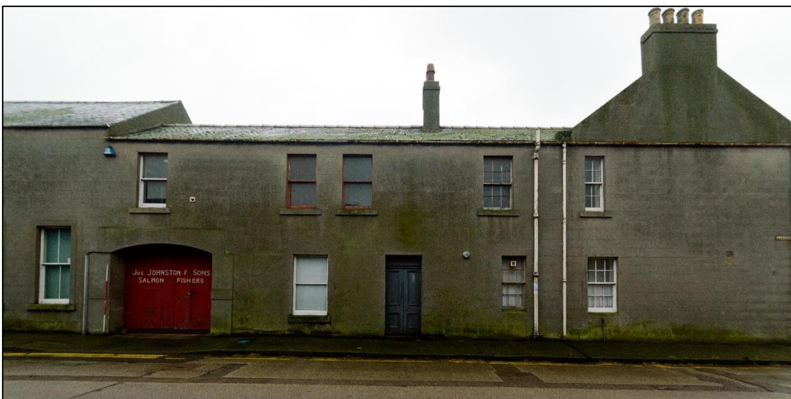
Illus 7 Nos 4 & 5, America Street, façade.
