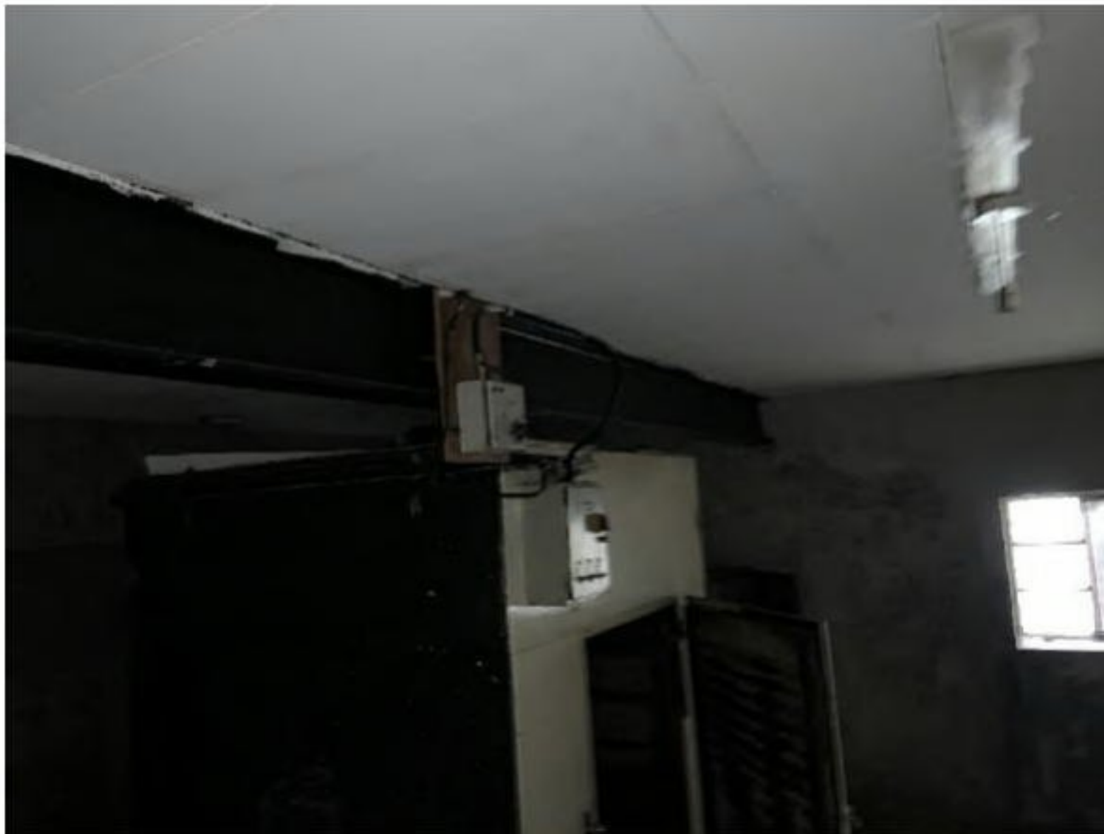
Photograph 3.09 - Old Workshop/Store – Steel Beams
