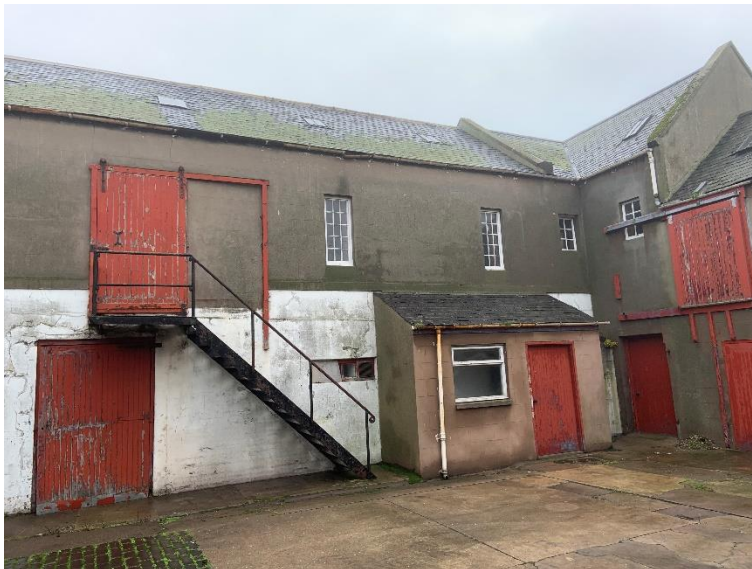
Photograph 3.05 - Old Workshop/Store – Quadrangle Elevation 2
