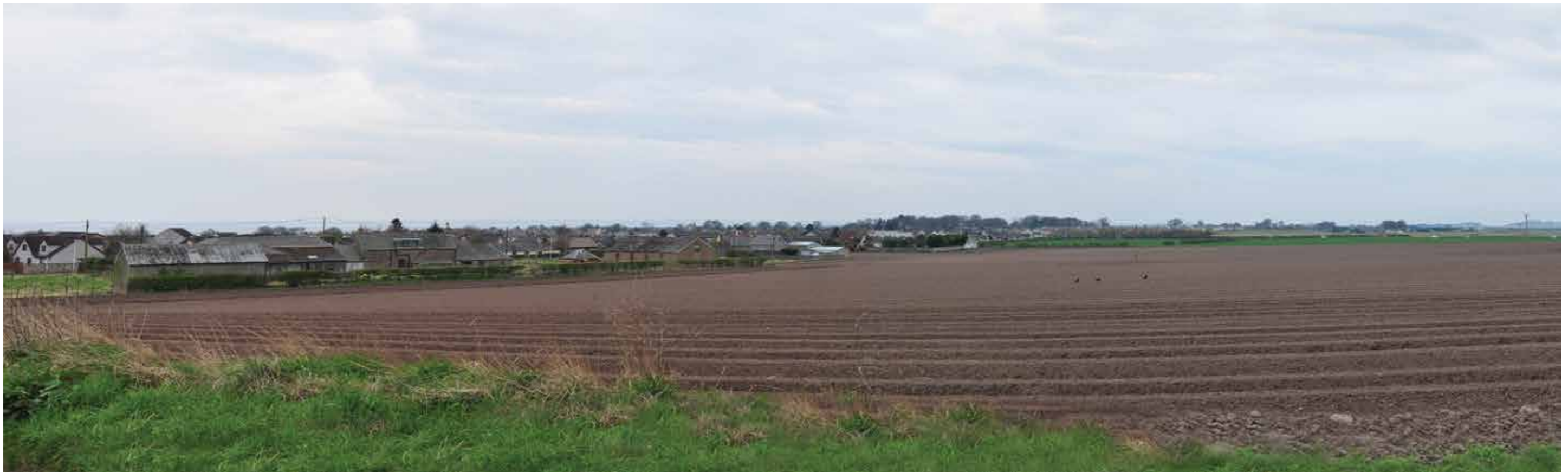
5.13 Approach from the North via U508-2 (From U508 Panbride Crossroads to A930)
