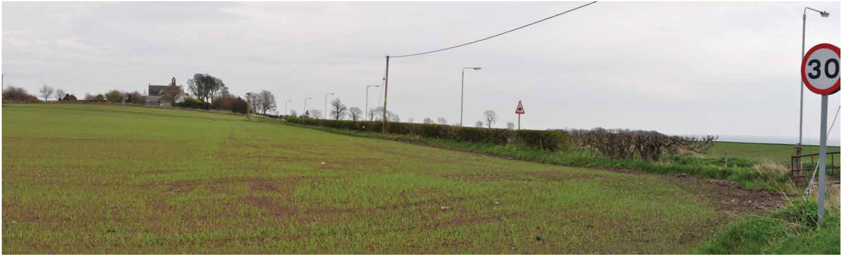
5.14 Approach from the North via U508-2 (From U508 Panbride Crossroads to A930)
