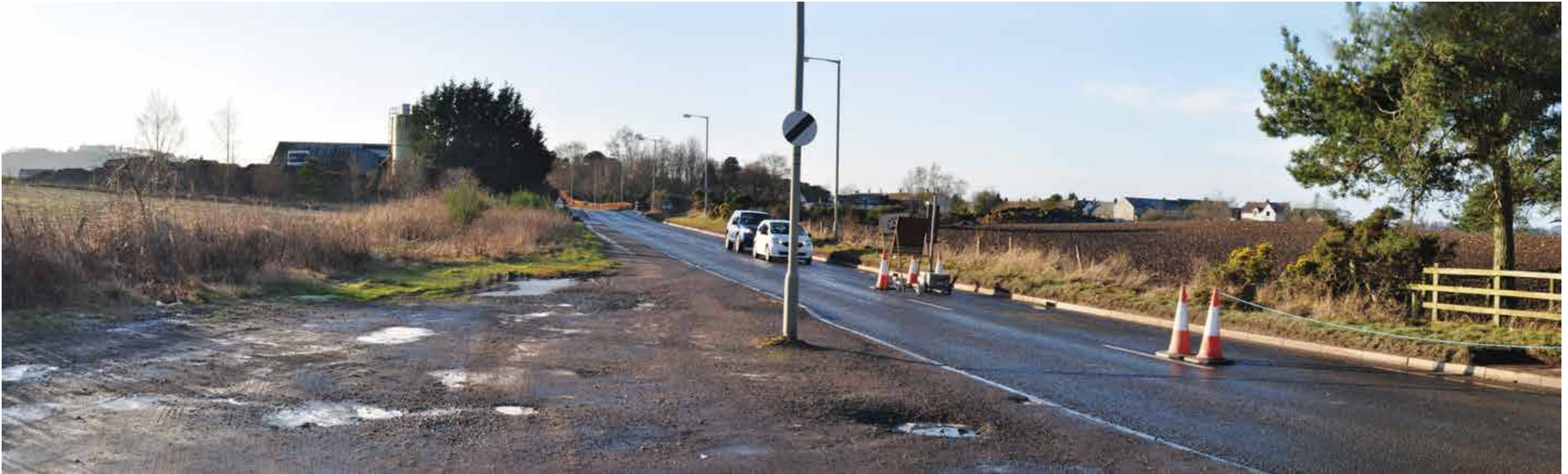
6.17 Approach from North-East via B9134 (Lunanhead Road)
