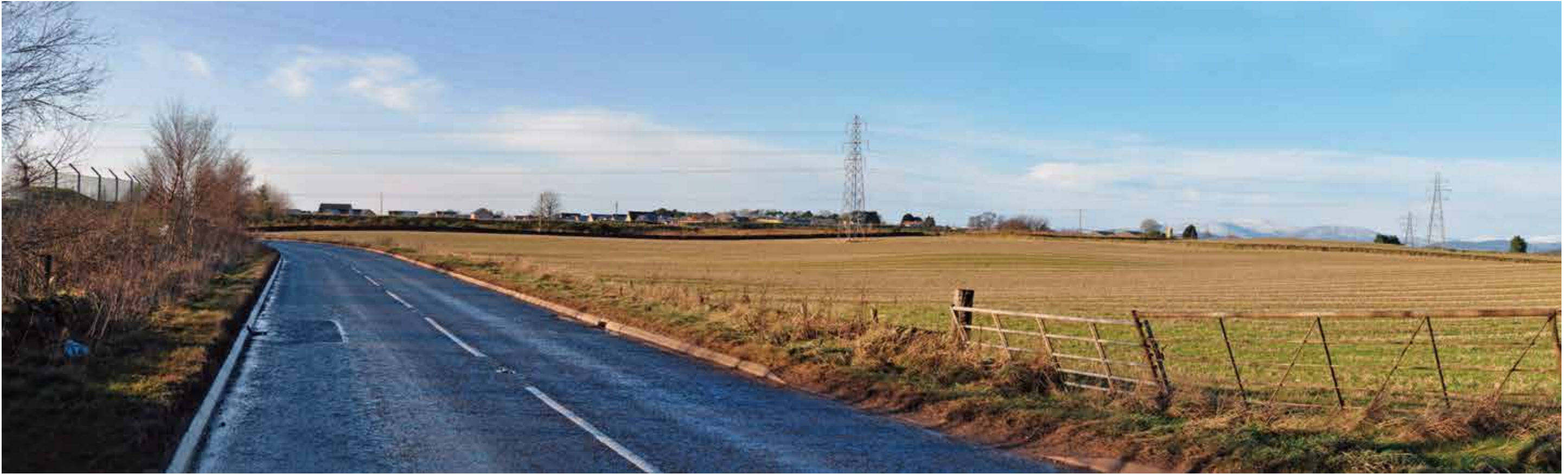
6.16 Approach from East via B9113 (Montrose Road)
