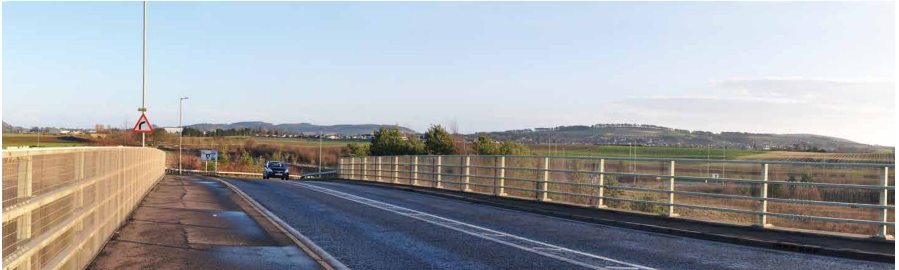
6.8 View from A926/A90(T) Junction
