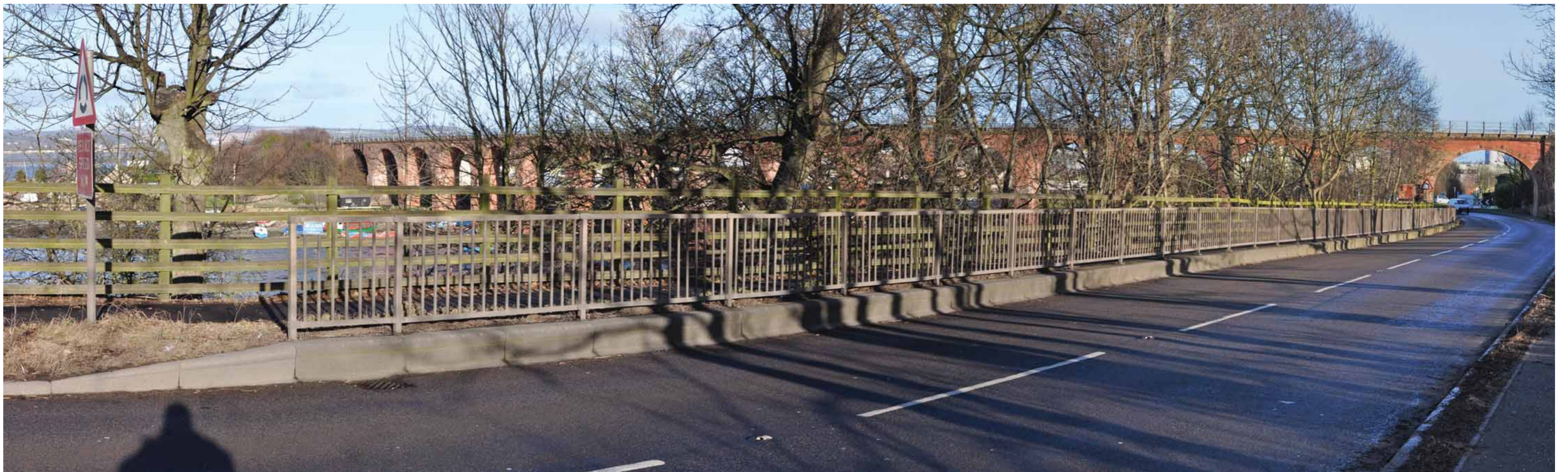
9.4 Approach from South West via A92 (Arbroath) ( click here to return to text )
