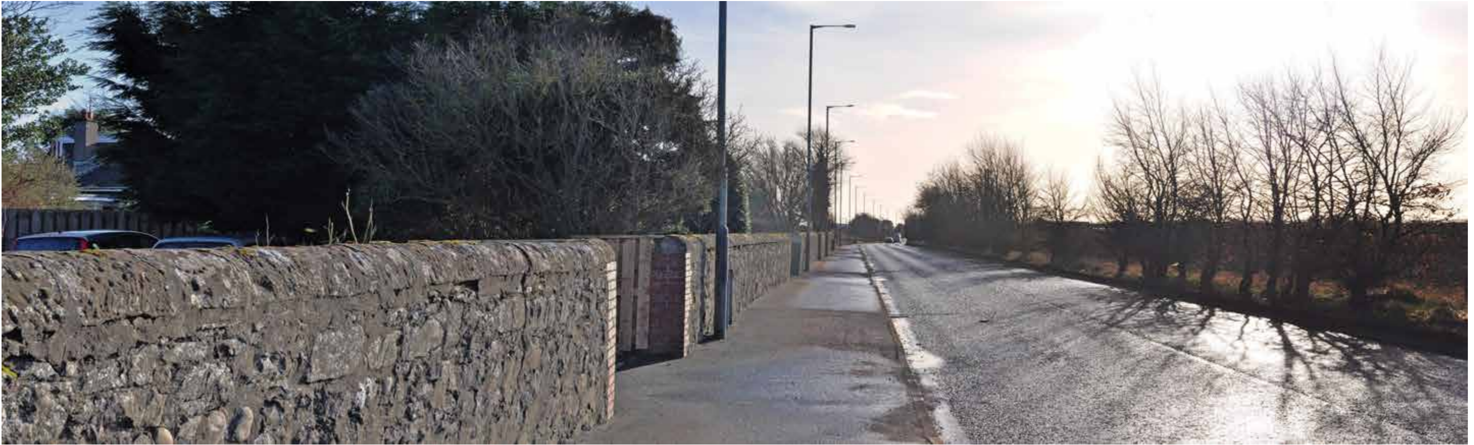
9.15 Montrose approach via A937 (Loan Dykes)
